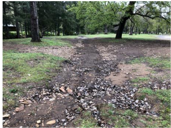
Reach A sheet erosion from overland flows 30/9/21
