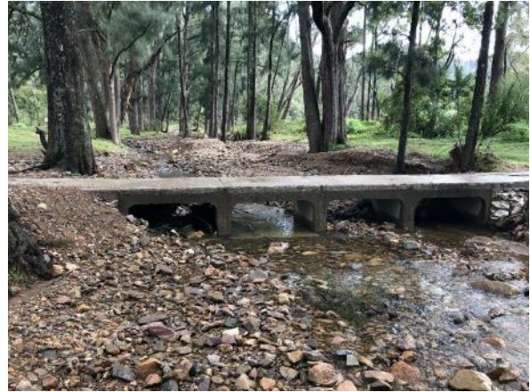
Reach A footbridge 30/9/21
