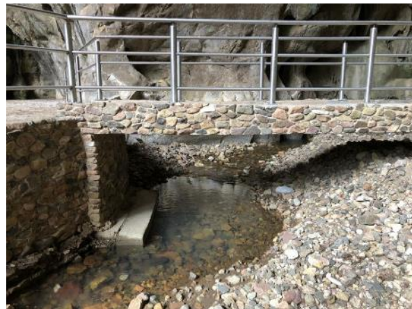
Reach D facing downstream at entrance 30/9/21
