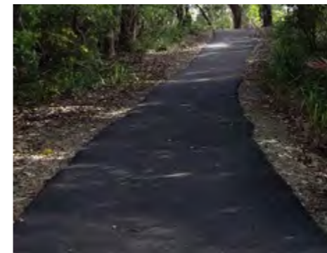
Typical asphalt path (class 1 access) (Source: EP NSW)
