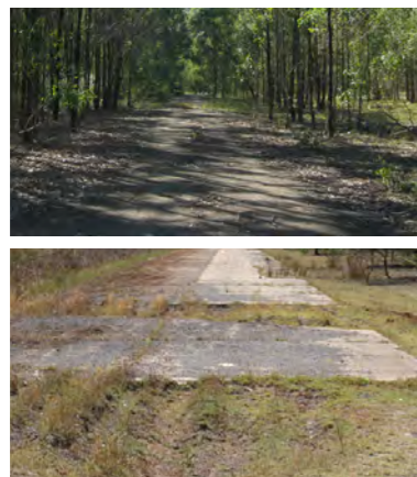
Site image: existing asphalt road (Source: EP NSW)
