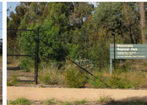
1.8m security fence (Source: EP NSW)
