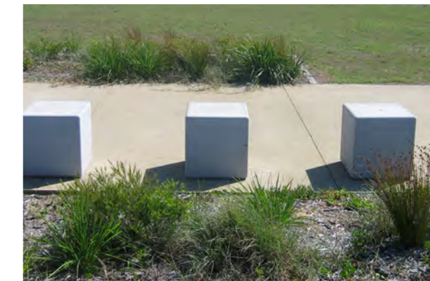
Site Image: Precast concrete bollards / seats (Source: EP NSW)
