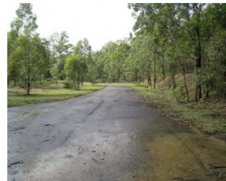
Site image: Existing concrete roadway (Source: EP NSW)
