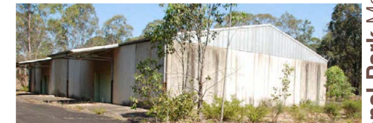
Reuse building 2 - NPWS workshop maintenance depot
