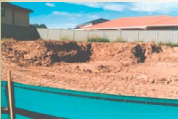
Soil exposed to the sun and wind may experience a higher rate of direct evaporation. Photo: DIPNR
