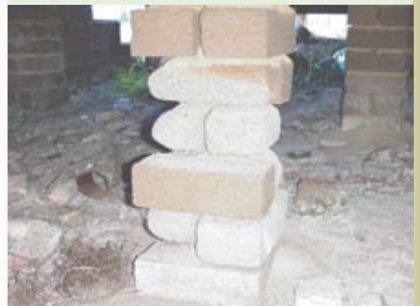
Bricks and mortar affected by salt and water action. Photo: DIPNR
