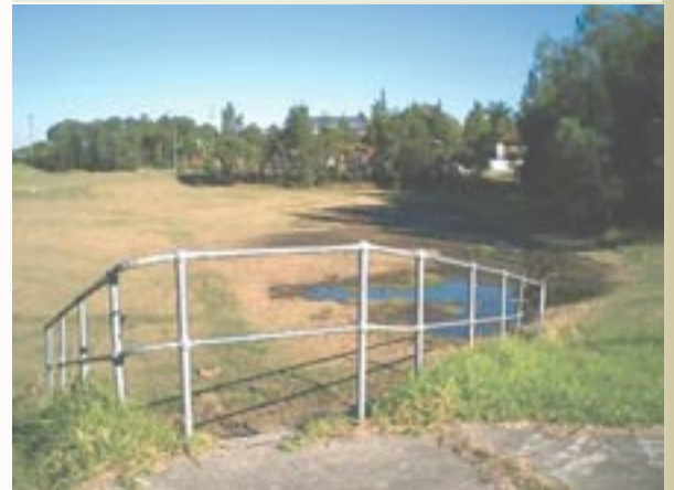
Waterlogged area that has a purpose as a retention basin. Photo: DIPNR
