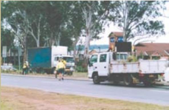
Maintenance being carried out by council. Photo: DIPNR
