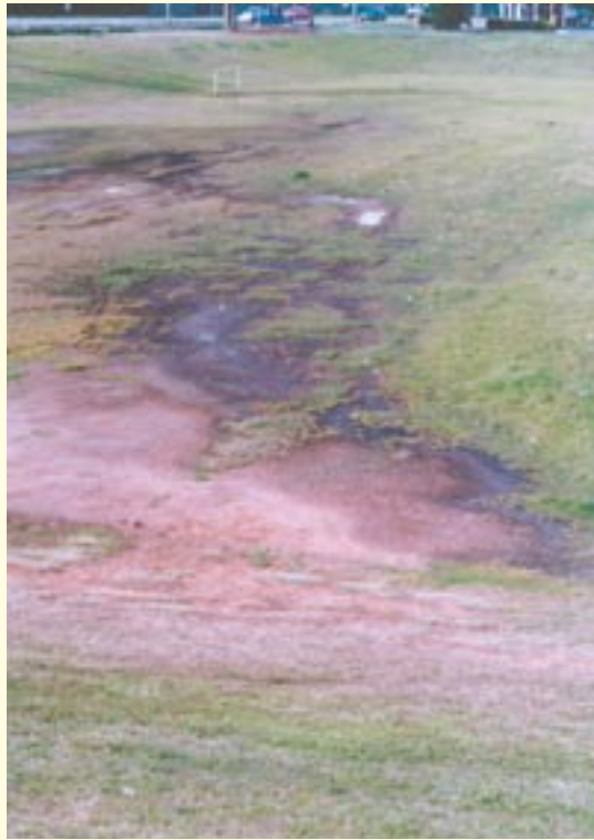
Waterlogged soil and bare patch in drainage/open space area. Photo: DIPNR
