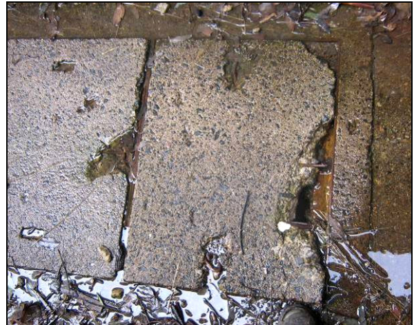
Figure 9 - Fallen grease level indicating water egress and cracked/broken lid leading to water ingress (photos Tom Pinzone/OEH)
