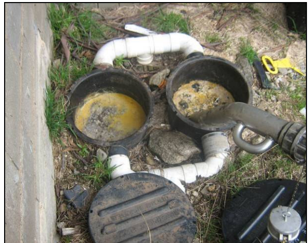
Figure 10 - Sewage contamination in grease trap and undersized grease traps (photos Tom Pinzone/OEH)
