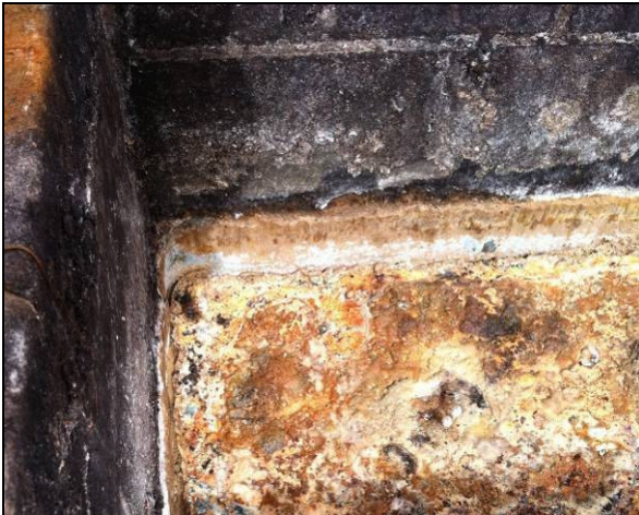
Figure 9 - Fallen grease level indicating water egress and cracked/broken lid leading to water ingress (photos Tom Pinzone/OEH)
