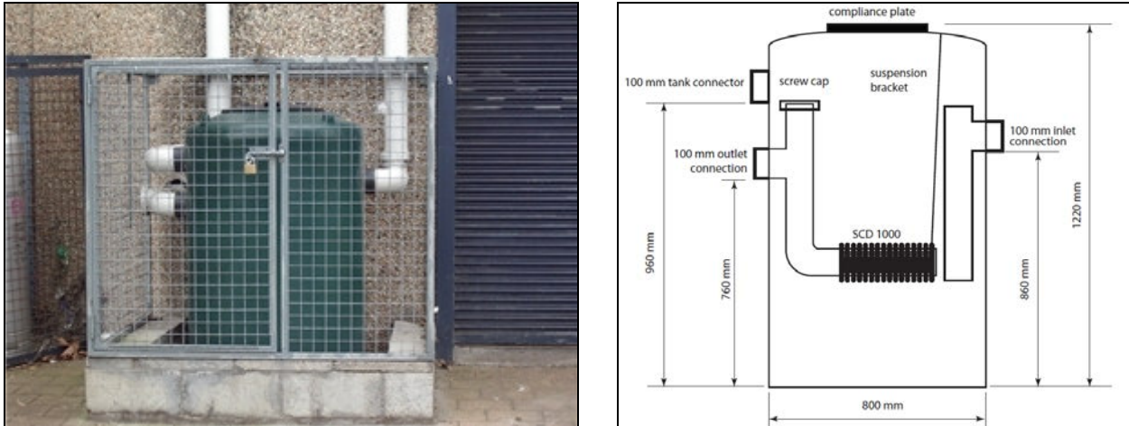
Figure 2 - Grease extractor and schematic diagram ( www.halgan.com.au )
