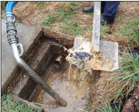
Figure 10 - Sewage contamination in grease trap and undersized grease traps (photos Tom Pinzone/OEH)
