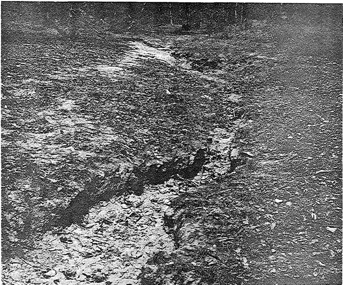
Figure 5. Minor gully erosion on Unit B soils.
