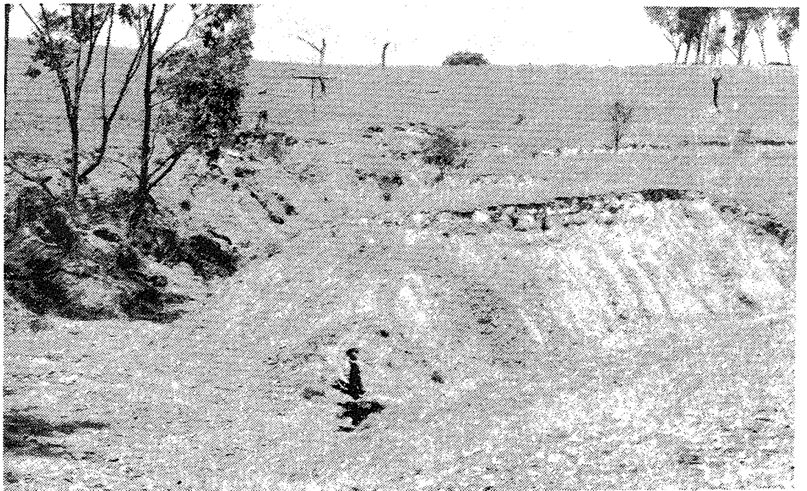
Figure 4. Severe gully erosion exists in the major drainage lines. This is a prime source of siltation now being observed and measured under rural conditions. Siltation will jeopardise proposed development and seriously reduce drainage capacities both in the Glenfield area and existing residential and industrial areas if not controlled.
