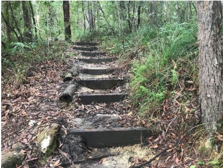
Plate 5. Steps on the Minyon loop track which will be replaced with stone.
