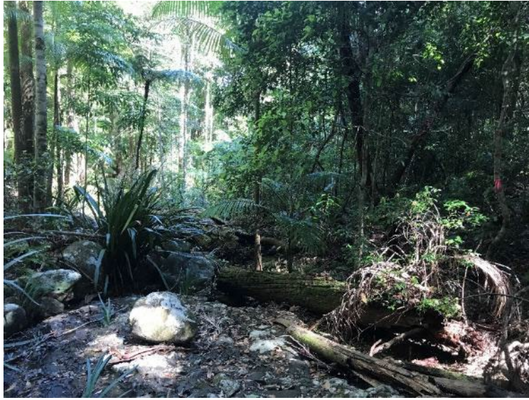
Plate 13. Watercourse crossing in Section 4 and use of natural rock shelf to minimise disturbance.
