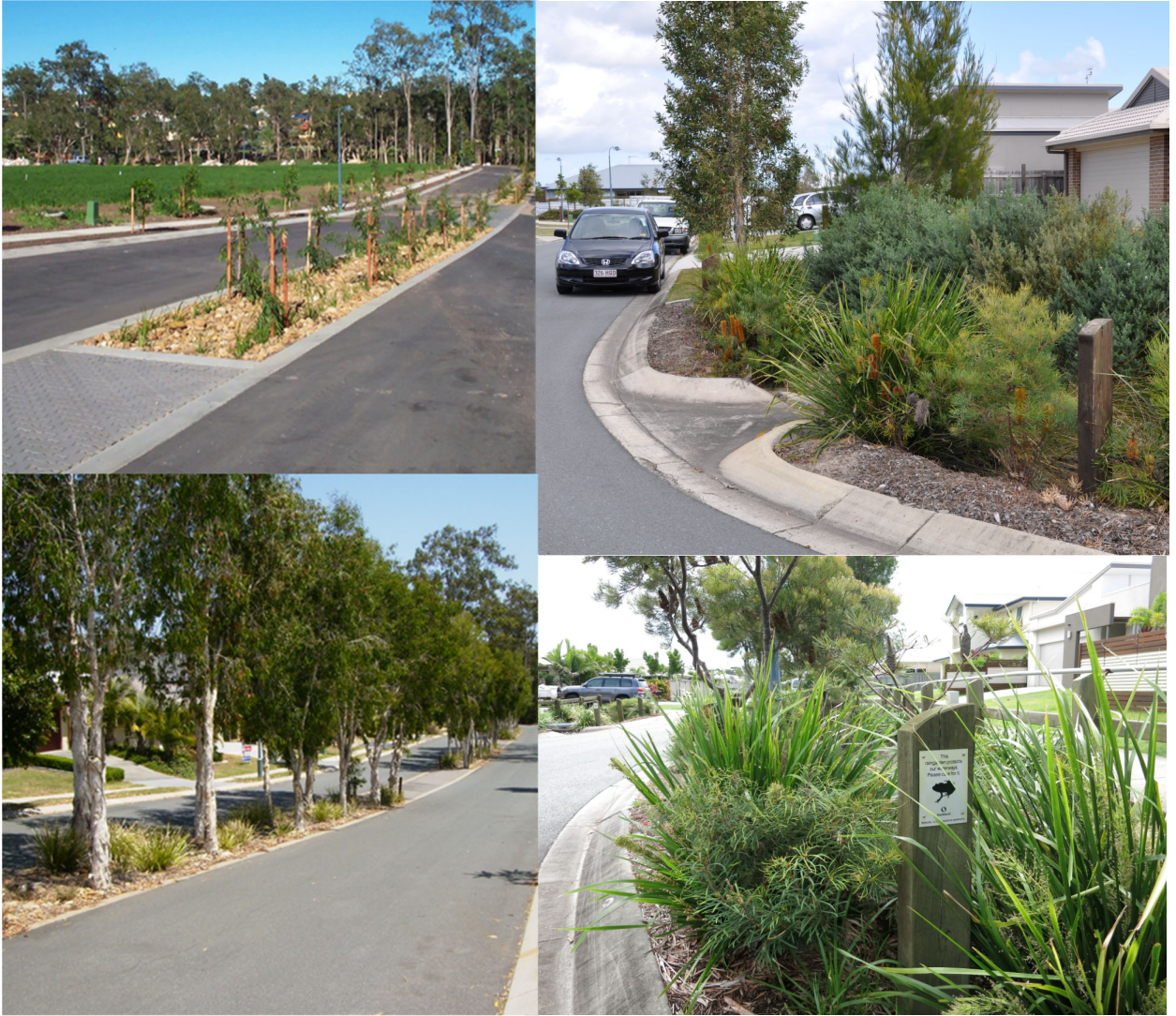
Figure 5-23 Example of streetscape water quality treatment and raingardens
