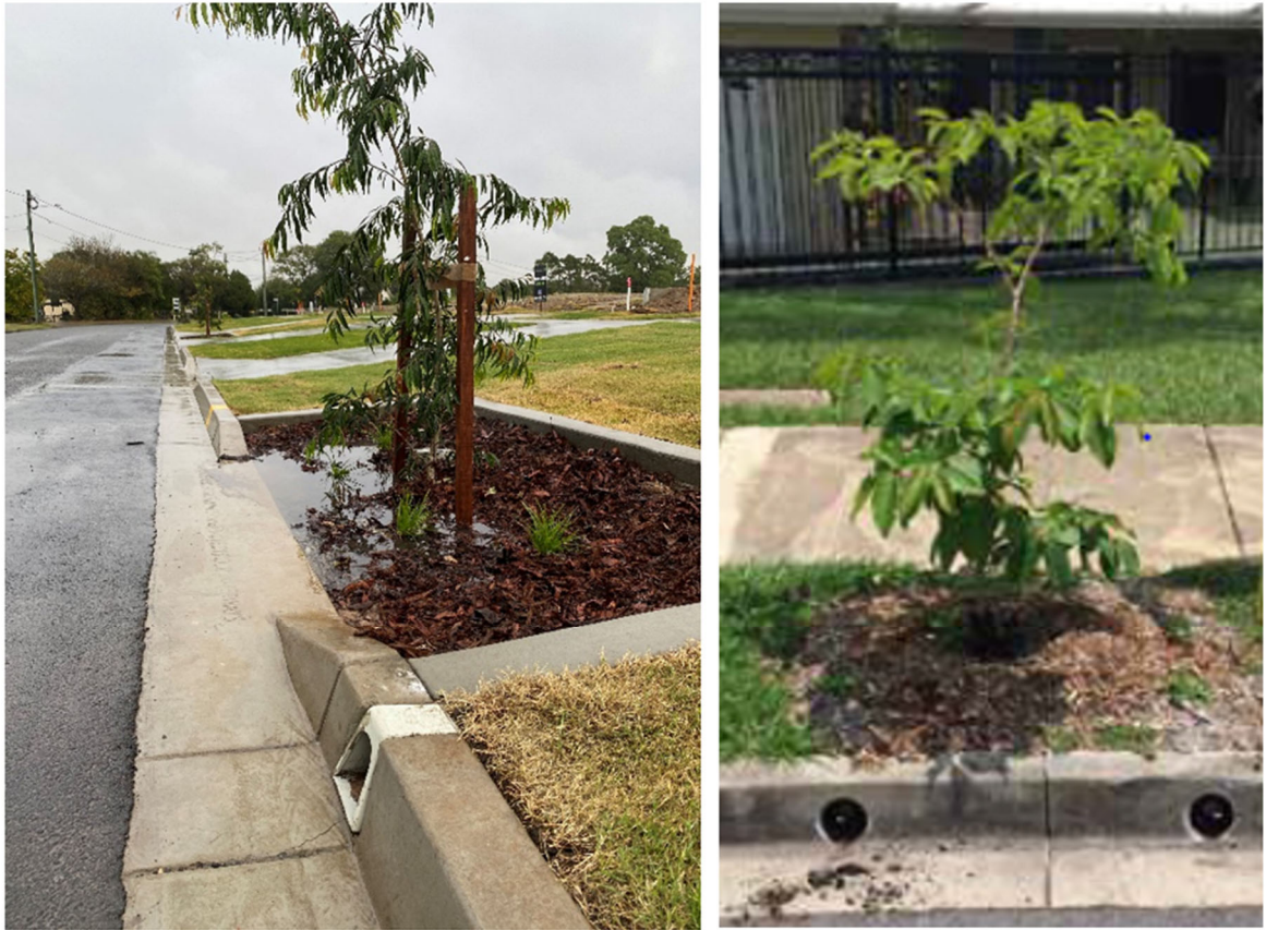
Figure 5-17 Examples of passively irrigated street trees
