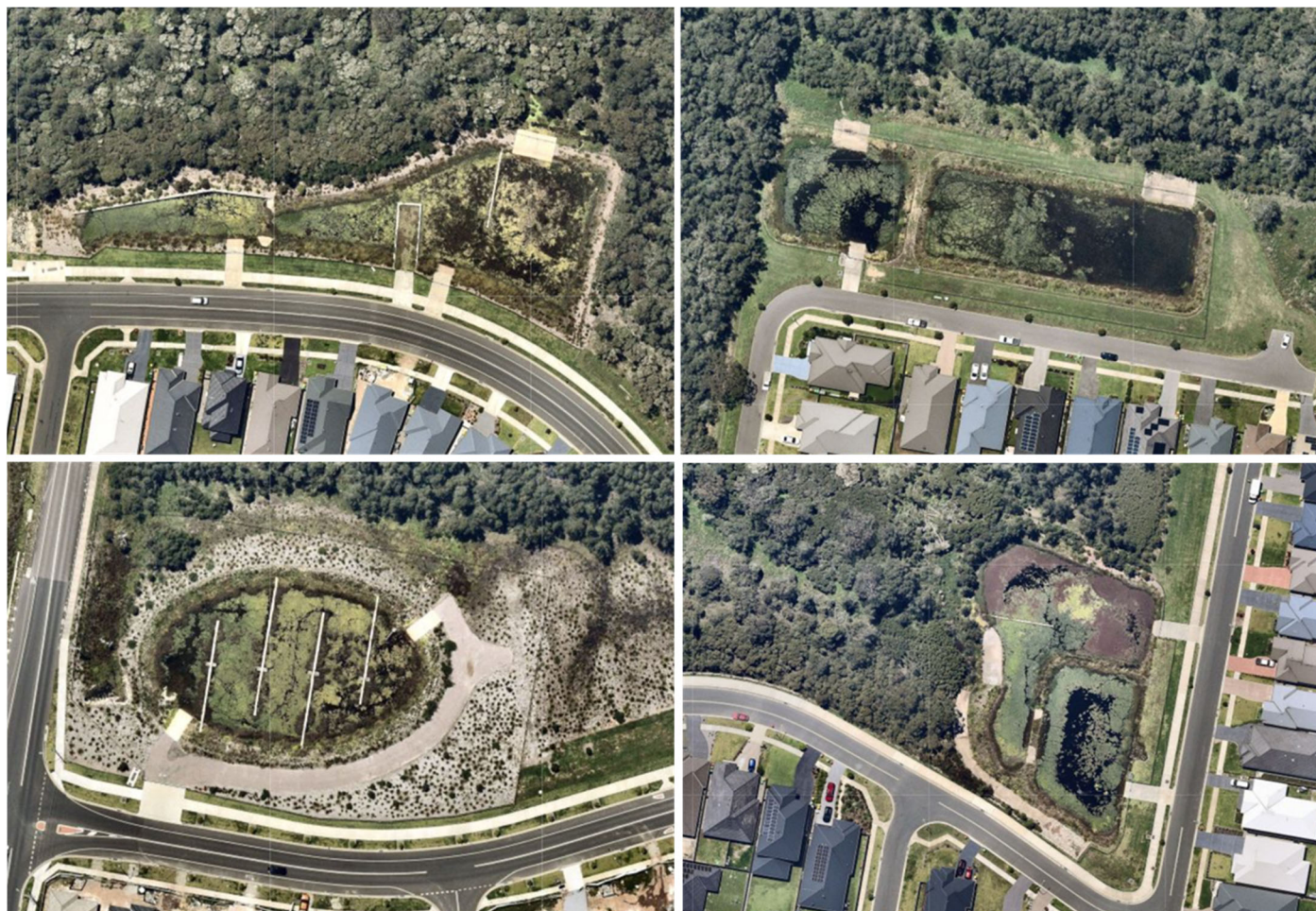
Figure 5-26 Example of eutrophic conditions in stormwater storage areas (4 November 2020)
