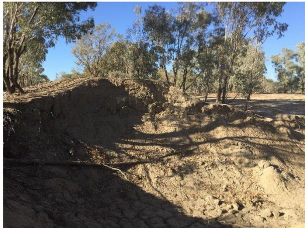
Figure 10: eroded section embankment
