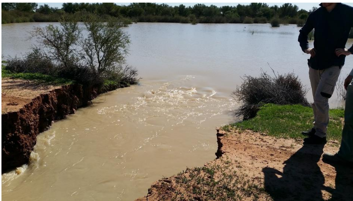
Figure 5-5: Breach in the eastern embankment allowing floodplain water to return to the Warrego River. Date: 15 May 2019
