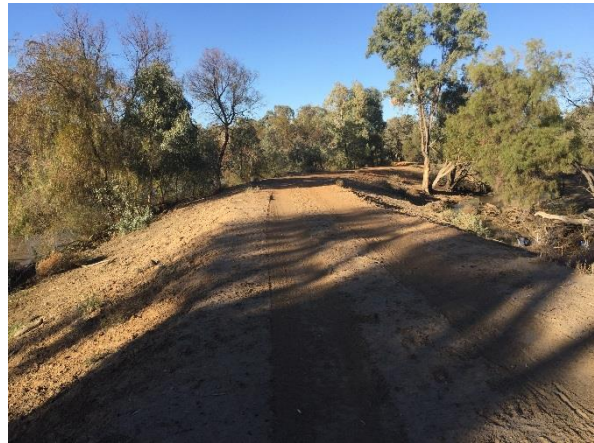
Figure 35: Boera Dam embankment
