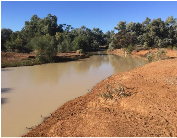
Figure 42: View of Homestead Dam embankment south of the homestead
