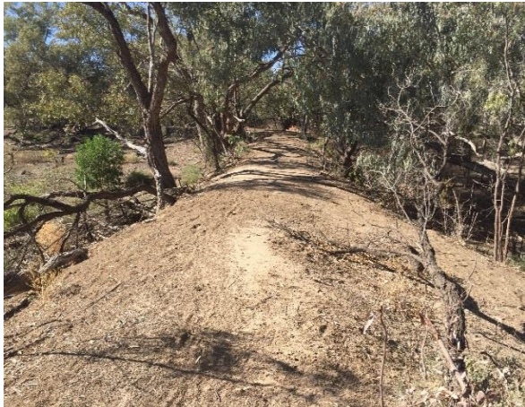
Figure 44: Embankment adjacent to the homestead
