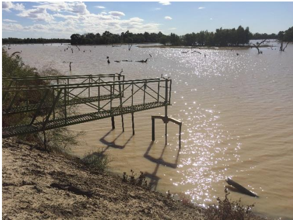
Figure 34: Boera Dam gates
