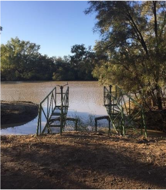
Figure 38: Booka Dam gates
