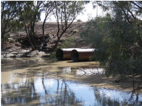
Figure 36: Infrastructure associated with Boera Dam
