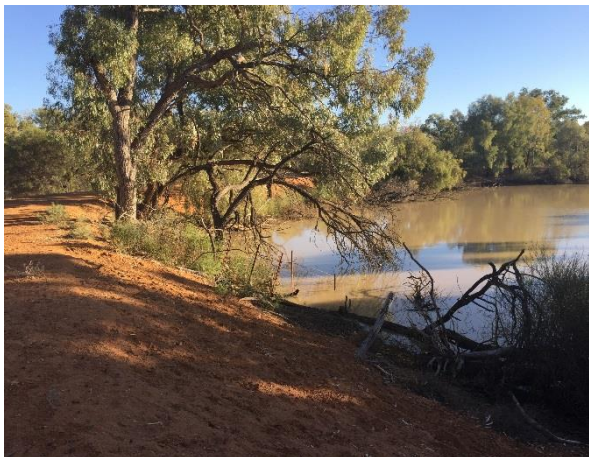
Figure 40: Booka Dam embankment
