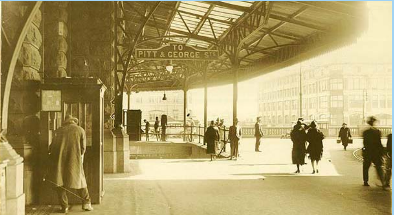
1924 image showing a skylight over the colonnade awning to the north-west corner of Central Station (Photo: NSW State Records)
