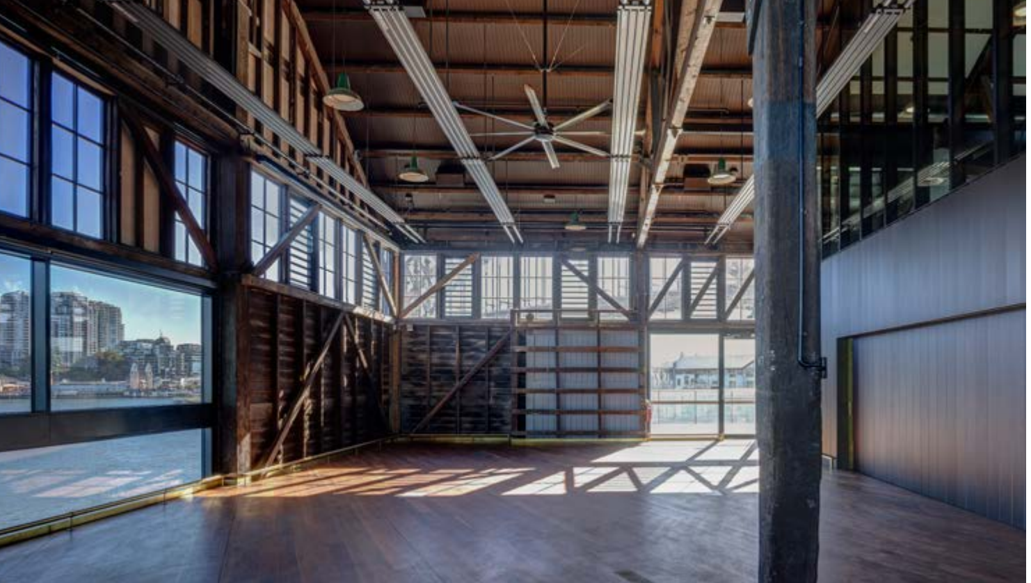
Glazed and louvred openings are used to provide natural light and fresh air to the Walsh Bay Arts Precinct. Ceiling fans and bar heaters are used to provide additional low-energy environmental control in the outer circulation spaces of the building (Photo: Brett Boardman for TZG)
