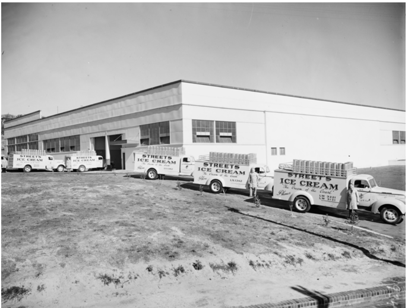
The Street’s Ice Cream factory in Turrella with light-coloured external walls demonstrates understanding of building colour and thermal performance – particularly important in keeping ice cream cold (Photo: Arthur Ernest Foster Collection, Mitchell Library, State Library of New South Wales)
