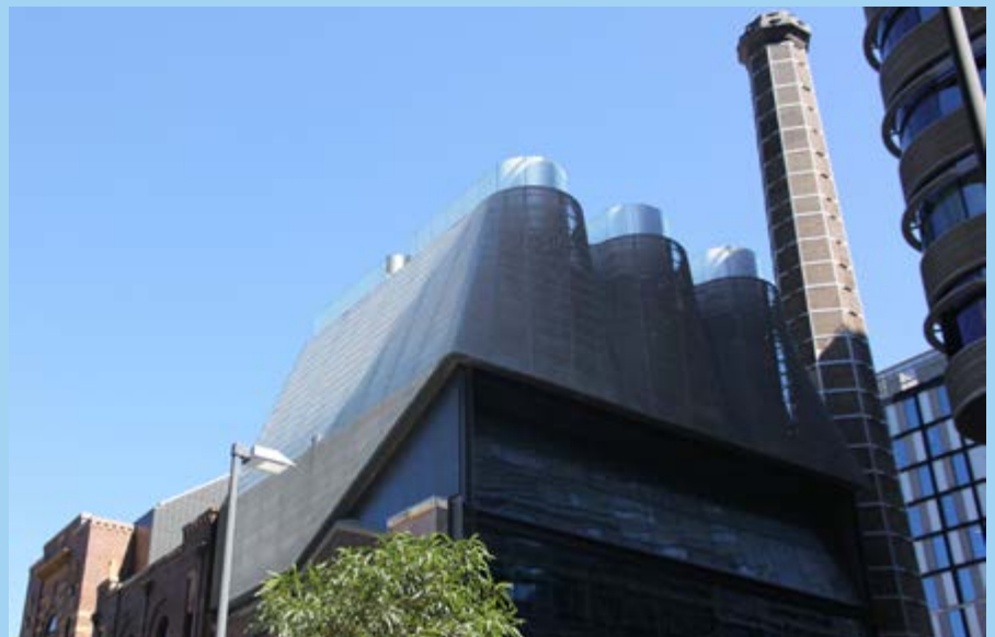
The former Kent Brewery adaptively reused to house the trigeneration equipment and cooling towers for Central Park, Sydney (Photo: Steven Barry/ Transport for NSW)
