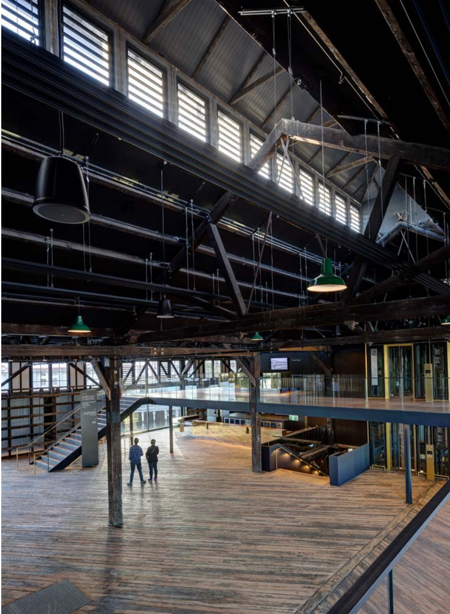
The ridge louvres of the Pier 2/3 building at the Walsh Bay Arts Precinct have been fitted with motorised actuators and connected to the BMS to provide automated opening and closing as needed (Photo: Brett Boardman for TZG)
