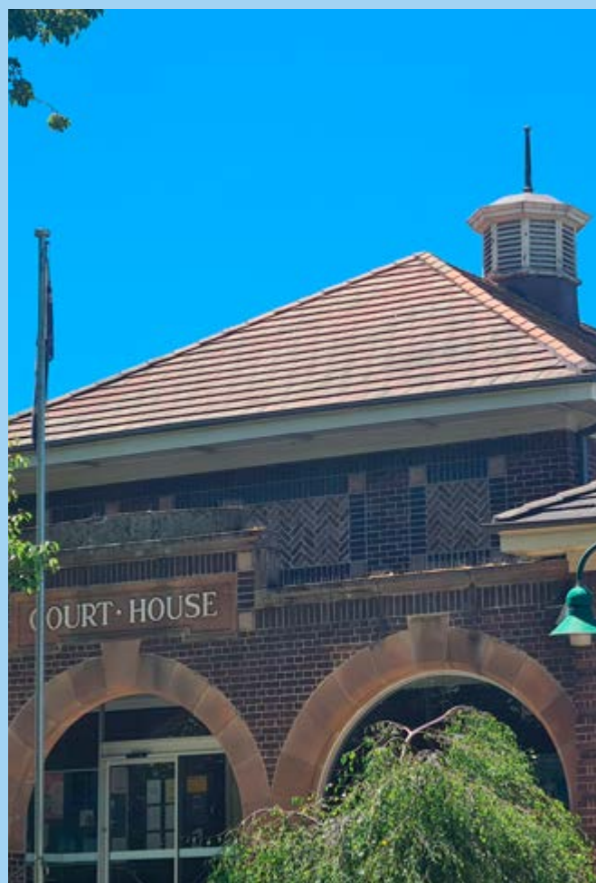
Moss Vale courthouse showing the central ‘turret’ or roof ventilator over the court room (Photo: Steven Barry/Transport for NSW)
