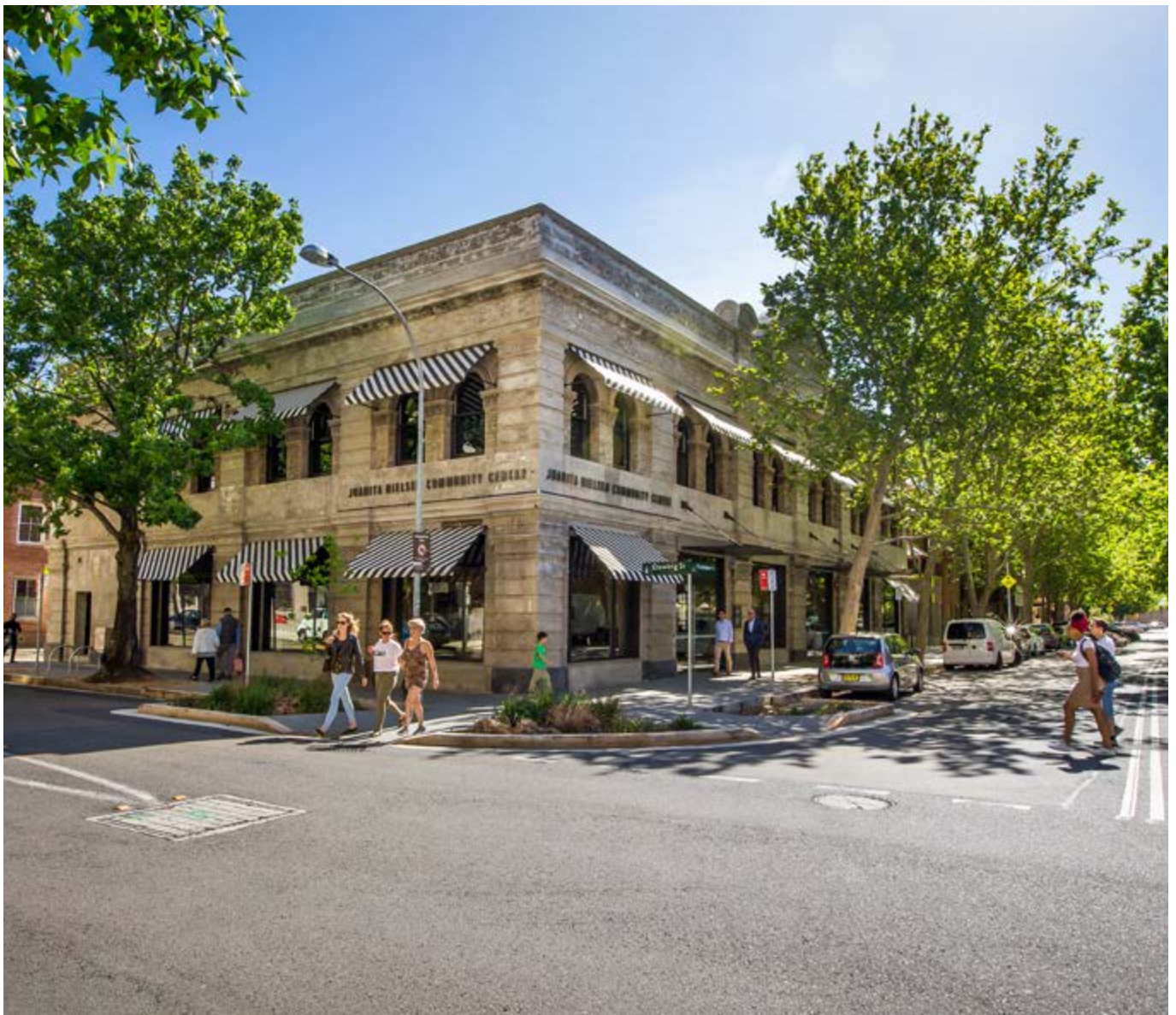
New external shading and canvas awnings were added to the Juanita Nielsen Community Centre in Woolloomooloo (Photo: Katherine Griffiths for City of Sydney)
