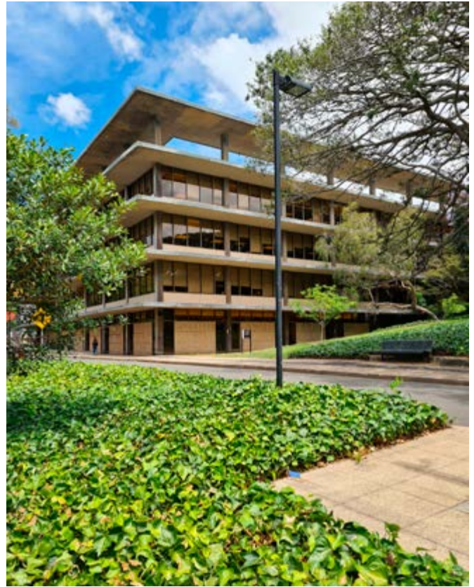
Fisher Library at the University of Sydney was completed in 1962 and features deep cantilevered concrete ledges which act as window hoods to the glazing below (Photo: Steven Barry/Transport for NSW)
