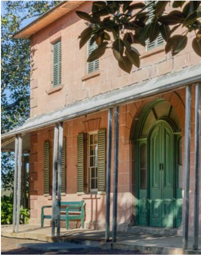
Rouse Hill Estate is a rural property in south-west Sydney and is managed by Museums of History NSW. The main buildings features external timber shutters to regulate light, temperature and natural ventilation (Photo: Katherine Lu for Museums of History NSW)
