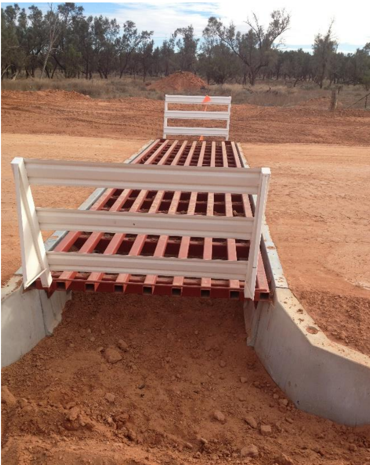
Figure 13: Example of an 8m-wide grid, rated for heavy traffic (up to 18 tonnes per axle), as proposed for Dunes Scenic Drive
