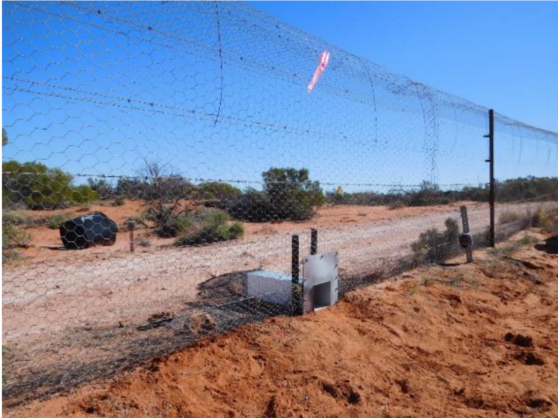
Figure 17: One-way gate installed within the Arid Recovery Reserve fence (Roxby Downs)
