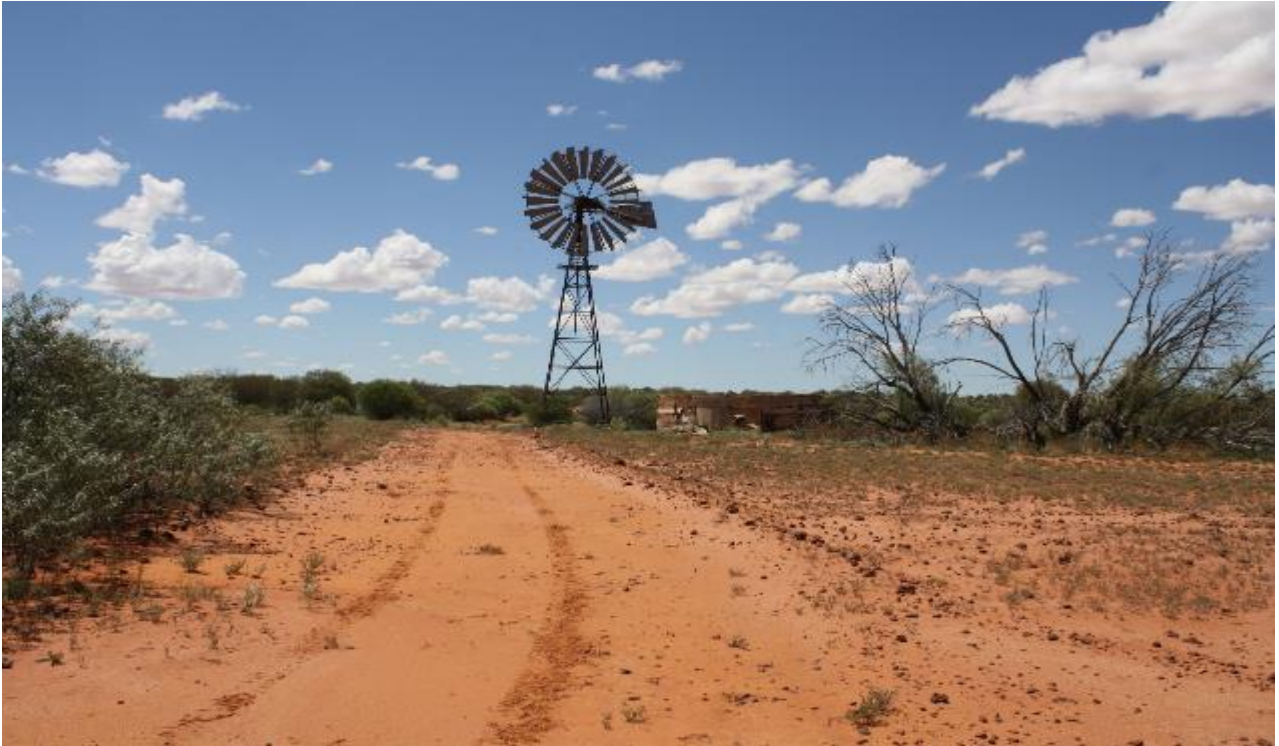
Figure 40: Defunct windmill, tank and trough at Corner Bore
