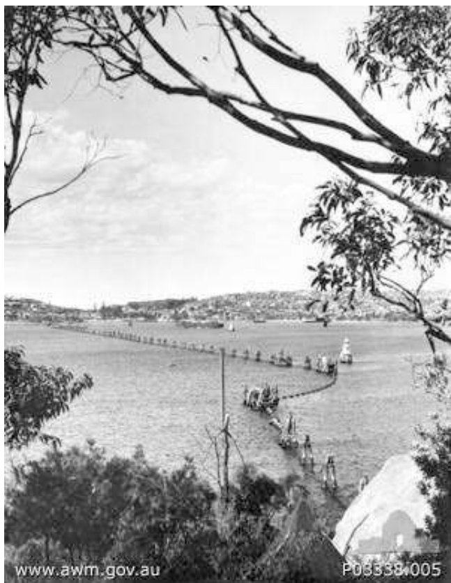
Figure 2.22. The Sydney Boom Defences Looking towards Green Point from Georges Head, 1942. (Source: The Australian War Memorial, id. P03338.005)
