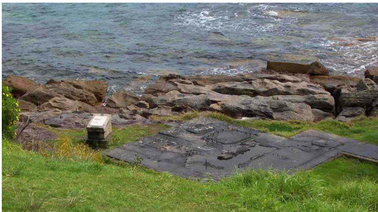
Figure 3.59. The foundations of Searchlight No. 4 (possibly also related to the boom net winch) are in the centre of the photograph alongside the memorial, which was erected in 1995 to record the World War Two Anti-Submarine and Torpedo Boom Net. October 2006
