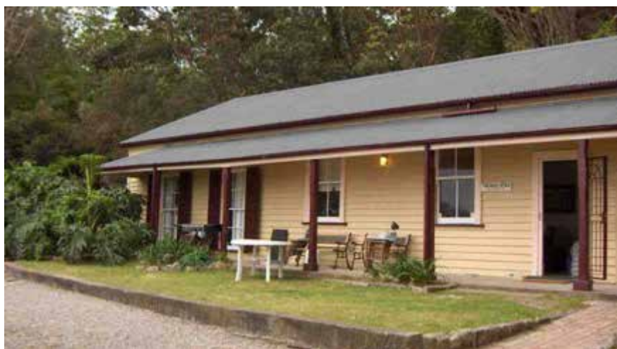
Figure 3.36. Constables Cottage. October 2006.
