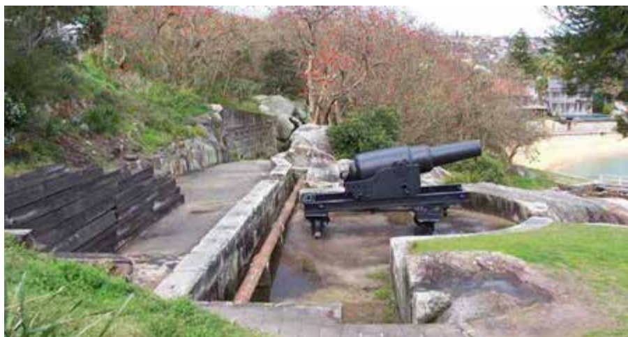
Figure 3.39. Looking south over the nineteenth century gun pit with Camp Cove in the distance. A 9-inch RML Mark V gun (on a carriage) relocated from elsewhere at South Head is housed at the pit. October 2006.
