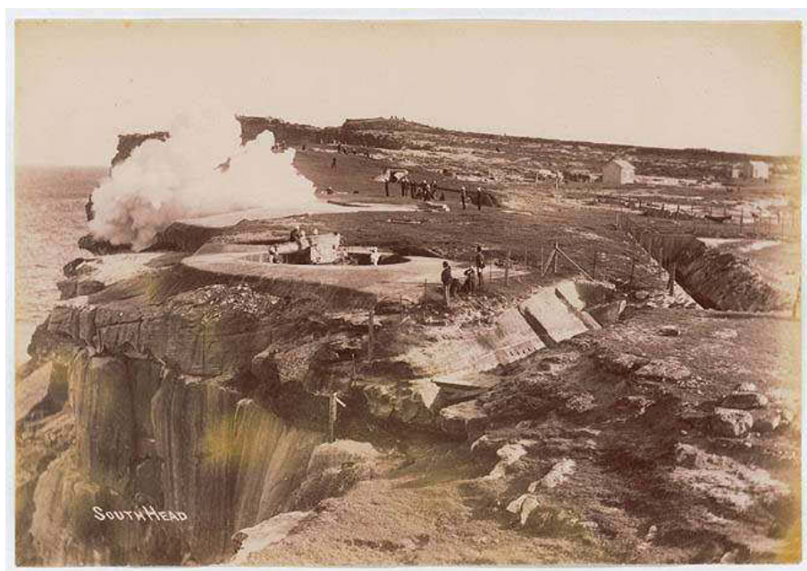
Figure 2.15. View of the South Head Fort c 1900–1910 (Hornby Battery), probably taken from inside the Hornby Light Tower, and showing the two gun emplacements (constructed 1876) inside the study area, and trench or moat to the rear of them on the right hand side of the photograph (see map above). It is possible that the smoke obscures the 6-inch HP ‘disappearing gun’. The 9-inch RML is in the foreground. (Source: State Library of NSW, Star Photo Co. - Unmounted views of NSW, [chiefly 1900–1910] PXE 711/23)
