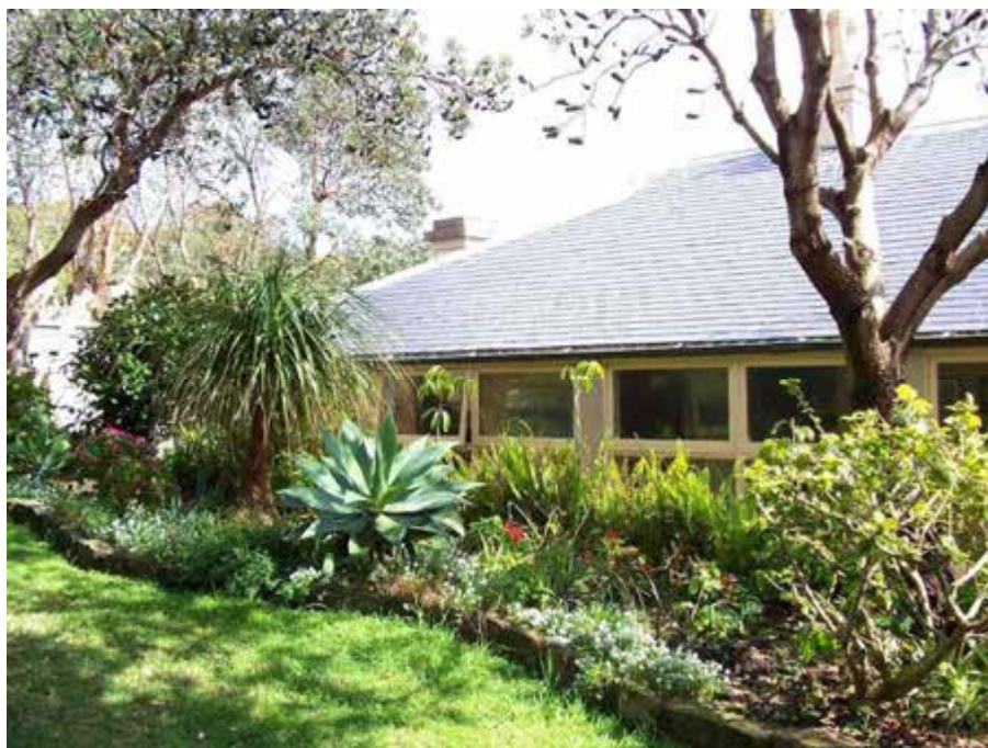
Figure 3.13. Looking at the south-east corner of the Assistant Lightkeepers Cottage with the cottages benched into the slope the verdant garden and showing the verandah enclosed in the 1940s and the recently installed slate roof. October 2006
