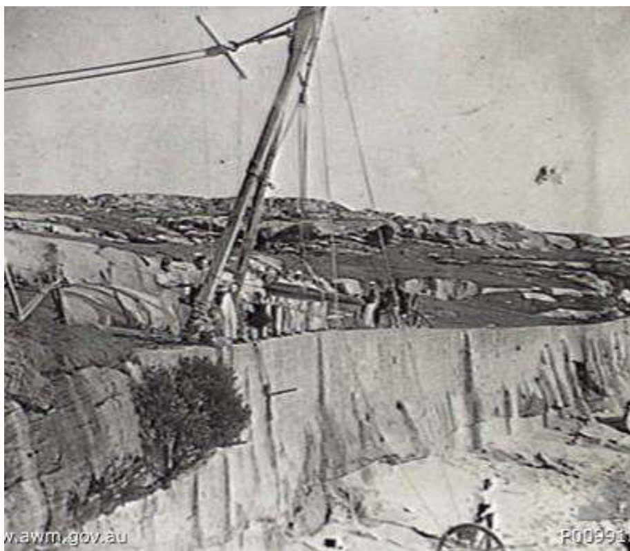
Figure 3.31: Sydney, NSW. 1898. Long course members of the south head NSW School of Artillery/Gunnery , after rafting a field gun to Lady Bay Beach, are shown using shear legs to lift the gun from the beach over the sea wall. Note the retaining wall built onto the natural bedrock (Source: AWM P991.074).
