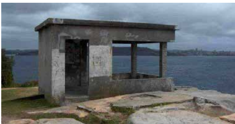
Figure 3.23. The WWII Searchlight Emplacement viewed from the southeast. October 2006
