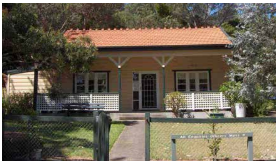
Figure 3.46. The front of the Workshop (now residence) from the west. October 2006
