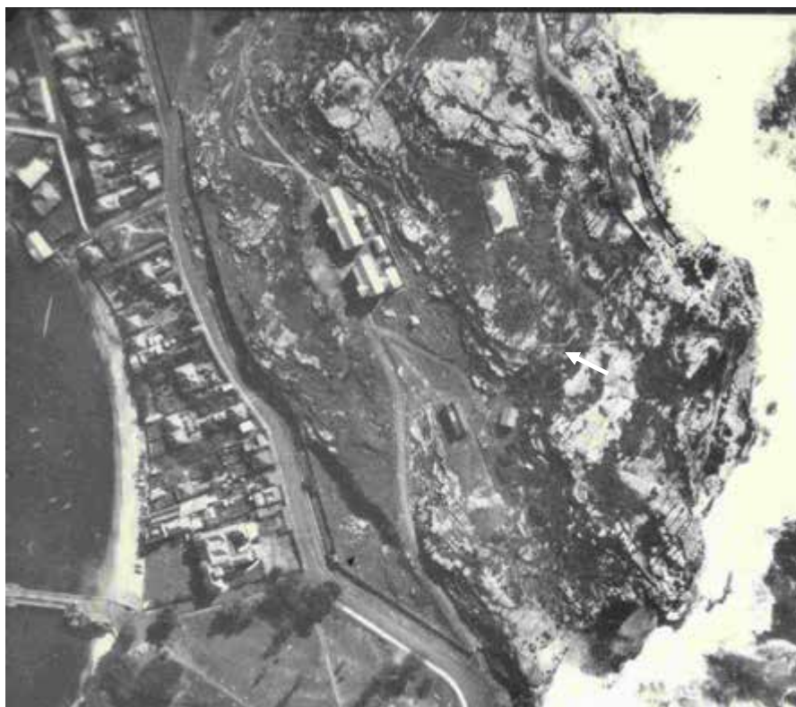
Figure 3.48. Part of the 1929 Aerial photograph showing Gap Bluff. The former Barrack buildings are clear, located in the north of the area and the Workshop is in the centre of the view with a vague line indicating the path to the Practice Battery in the northeast (top right). A wall bounds the area along Cliff Street. The remaining latrine is shown by the arrow. Source: DECC
