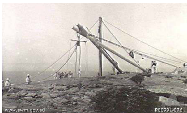
Figure 3.50: Sydney, NSW, 1898. Members Of The Long Course Of The NSW School of Artillery/Gunnery at South Head In The Process Of Erecting Shear Legs On A Cliff Top (Source: AWM P991.076).
