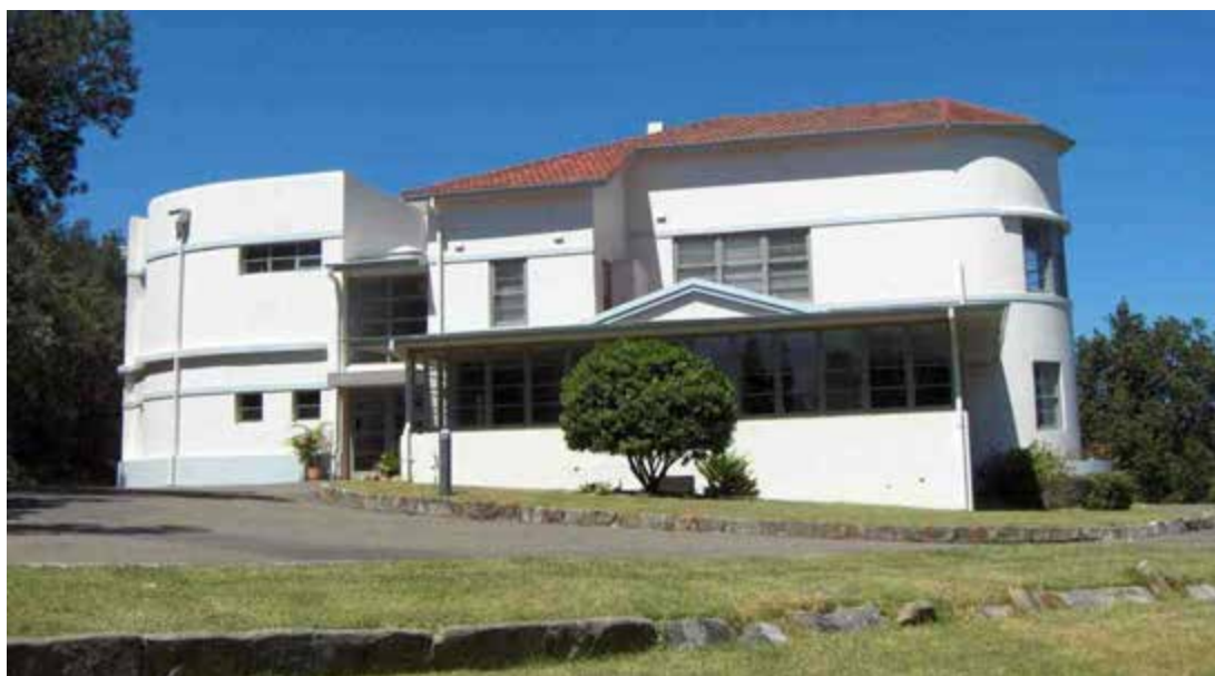
Figure 3.45. The exterior of the Officers' Mess from the southwest with the verandah in the foreground, the 1930s block behind (with its 1950s roof and the 1990s rear extension on the left. October 2006
