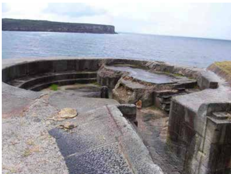
Figure 3.16. Looking north-east over the northern gun pit showing the 1876 work, the central pivot and the 1903 searchlight emplacement. October 2006.
