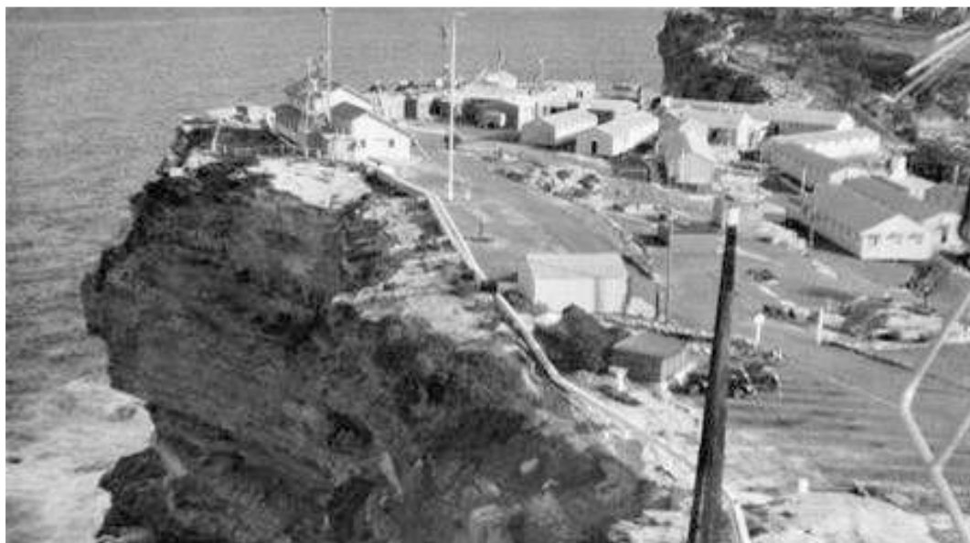
Figure 3.43. Part of a photograph taken of Gap Bluff showing the Royal Australian Navy radar training school in 1951. The buildings on the left at the top of the cliff are the Action Information Training Centre with a type 293 radar attached. Directly across the road are the maintenance and victualling areas with three mess buildings next to them. In front is the senior sailors mess, in the background is the Ratings mess hall and cook house and in between is the Ratings wet and dry canteen. The large buildings in the foreground are the Ratings living quarters and the small square building in front of them is the inflammable store. (Source: Australian War Memorial website www.awm.gov.au . Ref: P03815.006)
