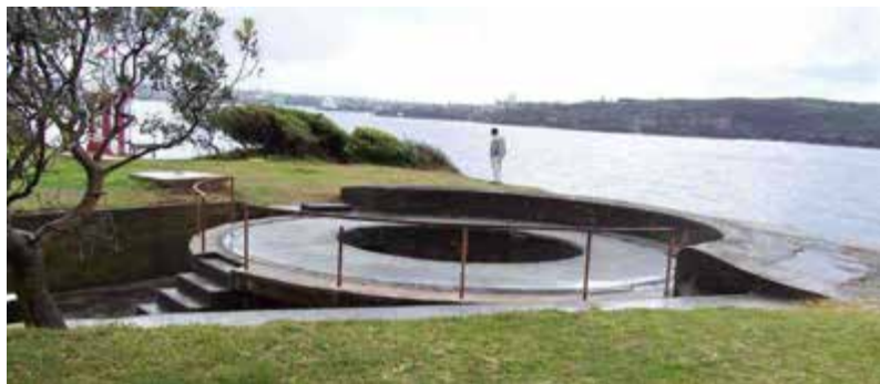
Figure 3.17. Looking north over the southern gun pit showing the 1889 and WWII works which substantially modified the emplacement to replace the 9-inch RML (fixed) gun with a 6-inch BL, MKV, and then with a 6-inch BL MKVII disappearing gun. October 2006.
