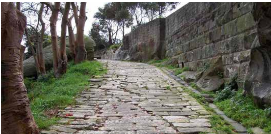
Figure 3.38. Looking north up the hill along the c1880s cobblestone road [IS 3.4] connecting the landing area and the Water Police at Camp Cove to South Head and the Hornby Light. The stone rifle walls flank the road on the east (right). October 2006.
