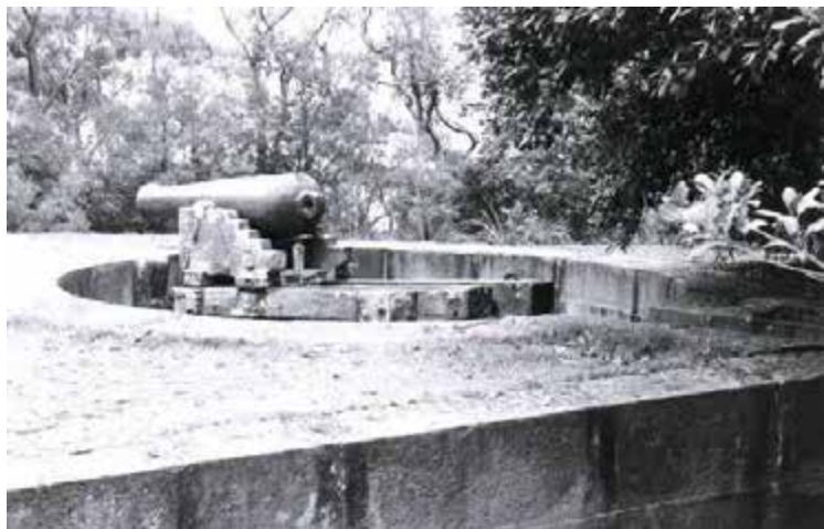
Figure 4.5. Part of the Bradleys Head Fortification Complex, Sydney Harbour National Park, Bradleys Head Road 1996. Photo from SHI 2060492
