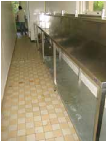
View of the commercial kitchen interior, at the rear part of building, associated with the function centre.
