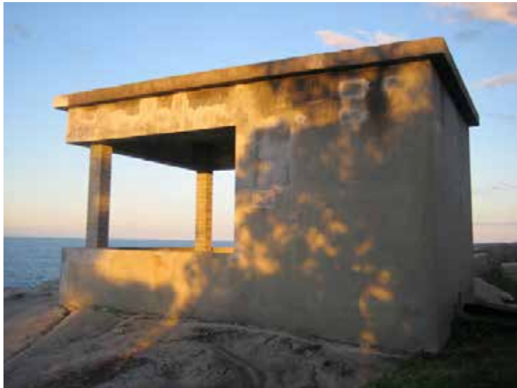
View WWII Searchlight Shelter, showing "remediation" work completed.
