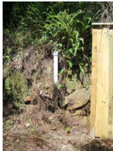
View of a drain pipe on cliff.
