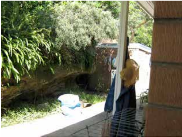
View of the rear yard facing the cliff with vegetation above. At the base of the cliff and running behind the outbuilding is a drain.
