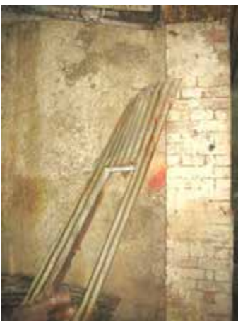
Former roofing sheets with skylight in the lightwell.
