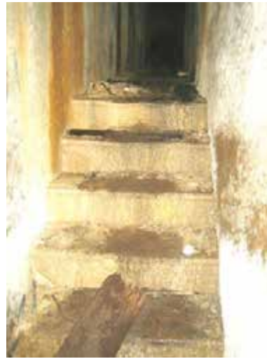
View of stone steps to passage possibly connecting to the Staff Room.
