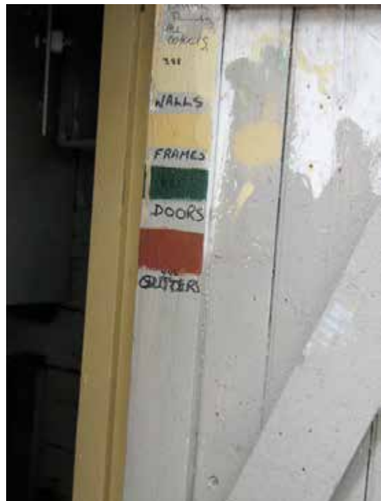
View of colour scheme, painted and described, on the rear of the storeroom door.
