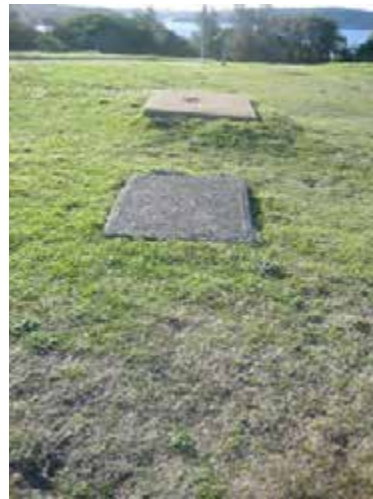
View of the two vent covers over the passage west of Shell Store, looking northwest from above.
