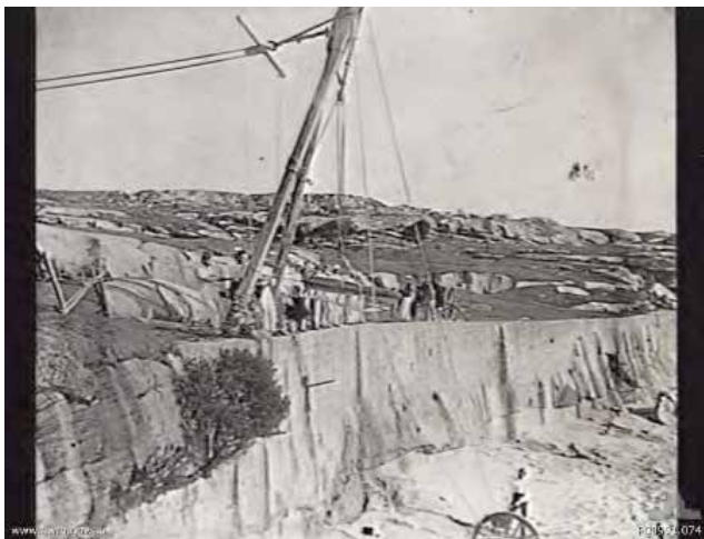
Using shear legs to lift a gun from the beach after rafting it to the beach, 1898. This image shows the low vegetation and the extensive stone walls. Source: AWM P00991.074.
