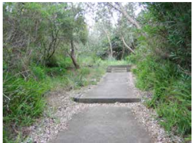
View of cement pathway and stairs in the Upper Gap Bluff area.
