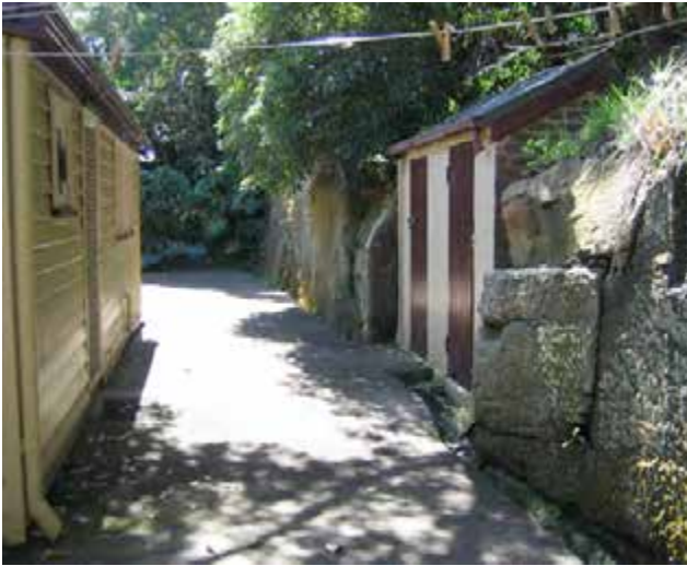
View of the rear space, with cemented paving, the down pipes discharging onto the paving on left side. The structure let into the cliff is the former WC's. There is a drain on the right.
