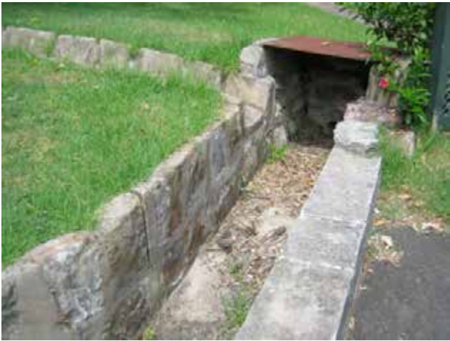
View of one of the stormwater drains, with stone walls.
