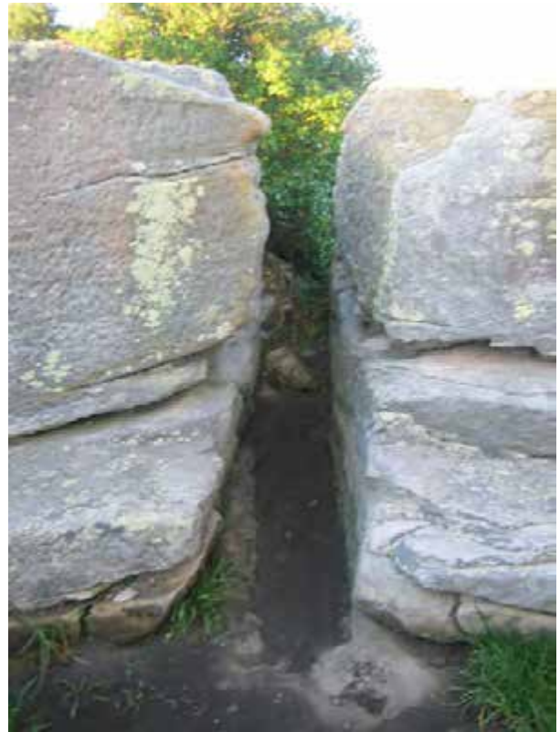
Drain from pit filled with silt and blocked by plant and roots.
