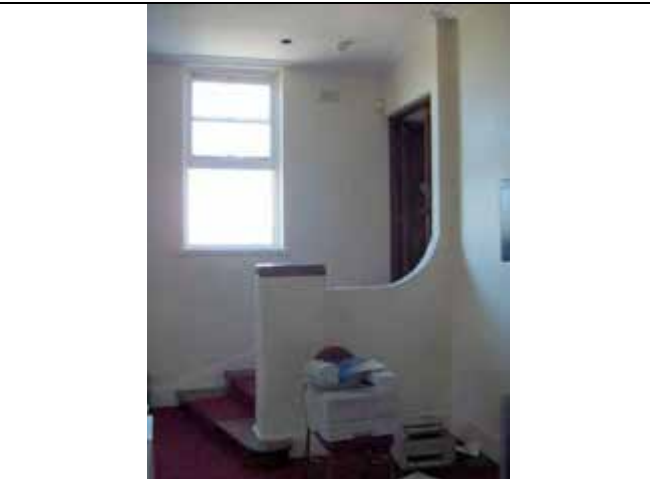
Interior of the First Floor Hall showing the half flight of stairs up to the former function rooms. October 2006
