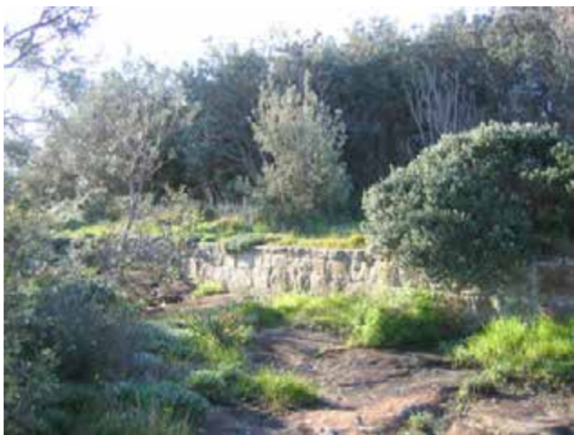
View of stone retaining walls.
