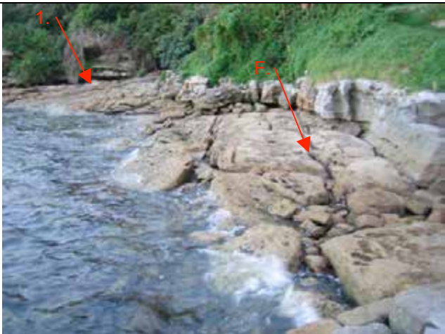
Current view of Camp Cove headland, showing the location of the remains of slipway (1.) The steps in the foreground where part of the wharf. The fissures (F.) are natural features not related to a former structure at that location.
