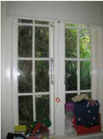
View of the casement windows (original), at rear.
