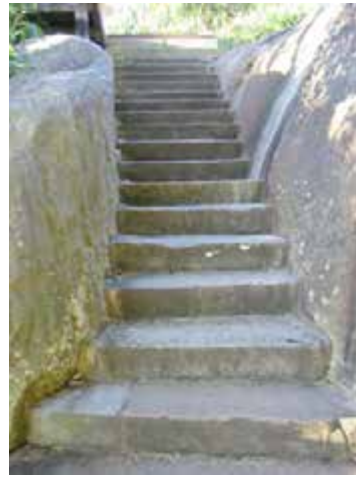
View of the early steps partly cut in rock, accessing the Lady Bay lookout, north of the beach, en route to Inner South Head.
