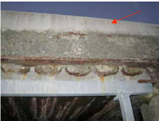
End view of Barlow rails supported by a new steel structure and new concrete slab over (arrowed).
