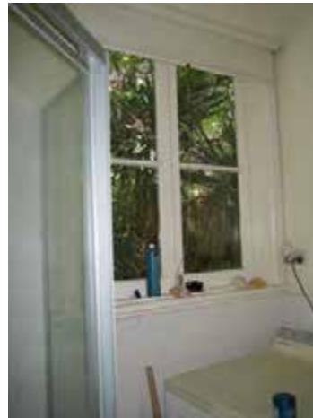
View of the casement windows (later added), at bathroom.
