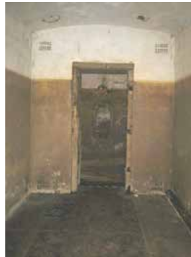
View of Magazine interior looking south to the door. Note the vents in the wall at the ceiling, left and right side, the marks on the thick bituminous floor and on the ceiling are of structure for earlier shelves. The marks on wall are the former water level when the area was flooded, it is not paint.
