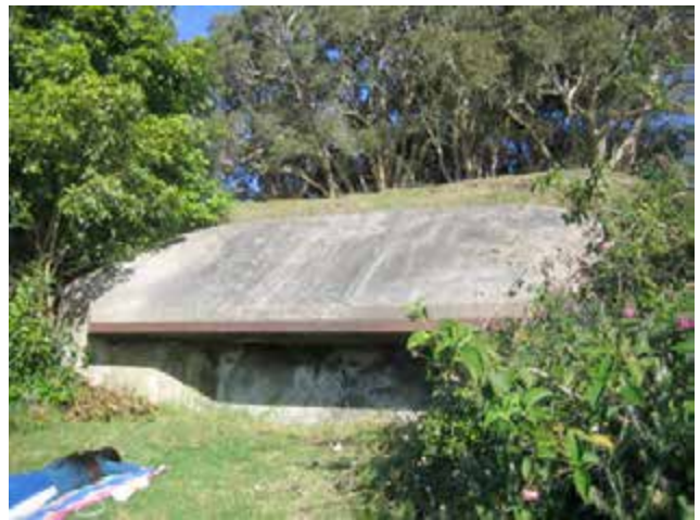
Closer view of the above ground remains assumed to be part of the Submarine Miners Firing Station. The observation opening is blocked.
