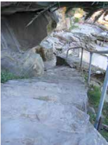
View of the steep stairway and handrail at access to Lady Bay Beach.
