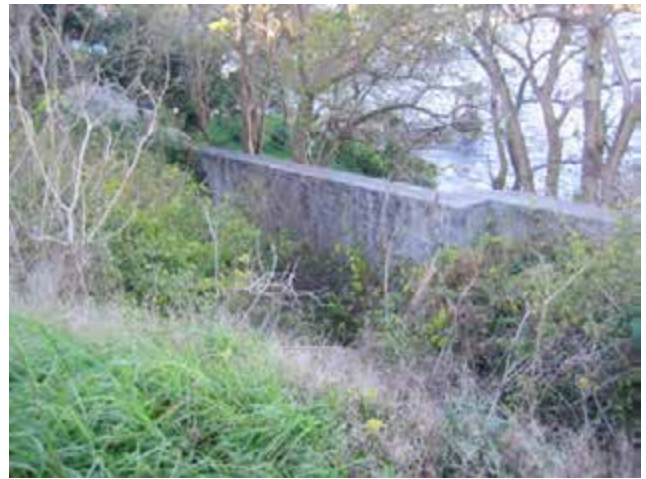
View of the rifle walls from above the Cobblestone Road. Note Lantana and other weeds.
