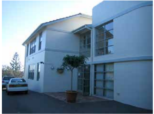
View of the rear (east) elevation. Addition to the building is on the right side of picture. Glazing of larger windows is fixed, precluding natural ventilation.
