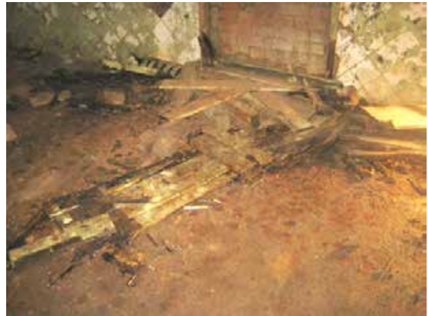
Remains of the door, now bricked up, in the south wall.
