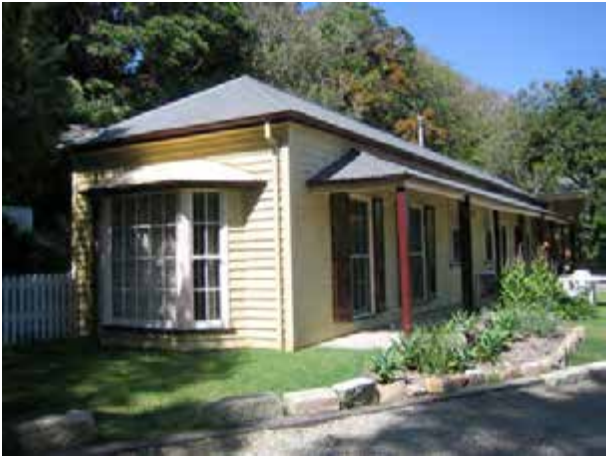
View of the building looking south. The bay window and full length windows are the 1950's addition.
