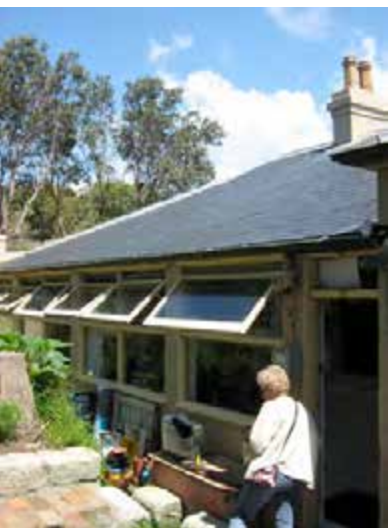
View of the east verandah showing altered enclosure.
