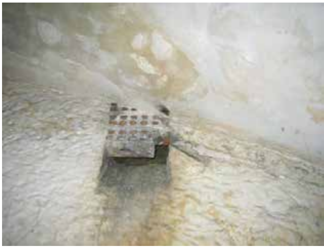
One of four vents to the exterior (at ceiling).
