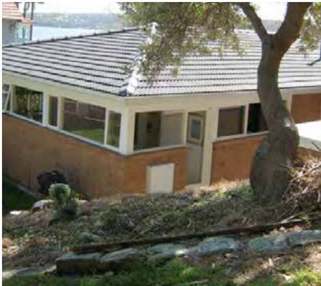
View, from the elevated rear yard, of the building tiled hipped roof looking northwest towards harbour. The area, behind the photographer, is generally weeds.
