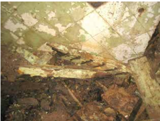
Remains of former door in the south wall showing detail of frame for louvres over the door.
