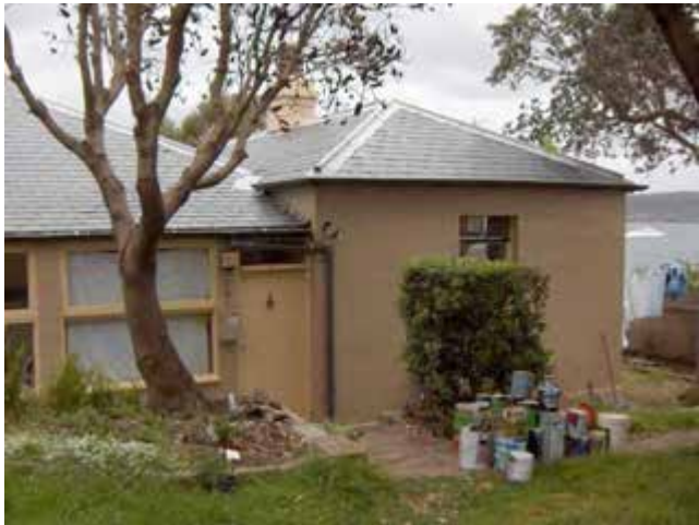
The east Assistant Light Keepers Cottage looking from the south east with the 1857 work with its filled in verandah on the left and the hipped roof 1878 extension on the right. October 2006.
