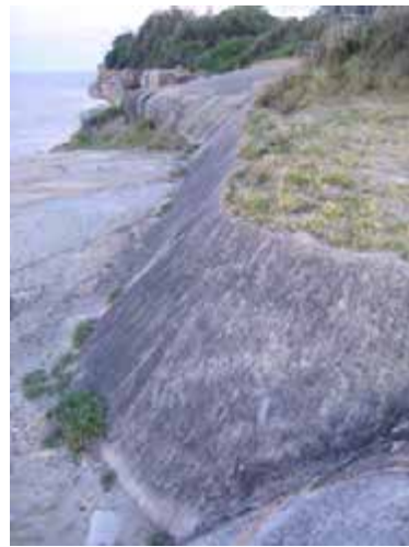
View of part of the concrete embankment forming edge of gun emplacement.
