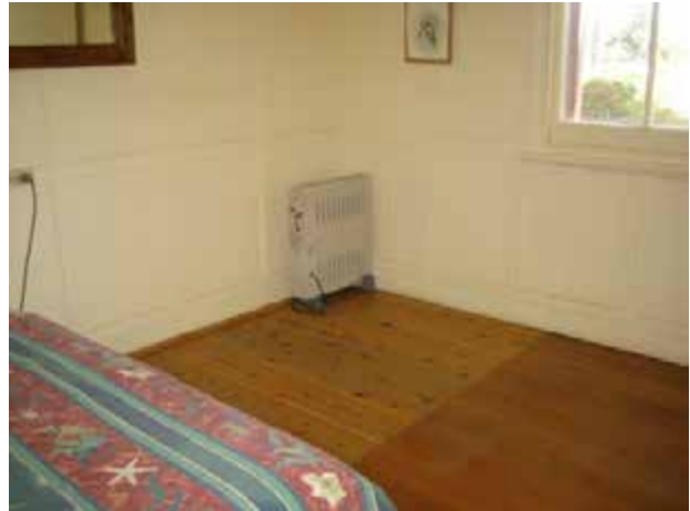
View of bedroom with partially replaced floor.
