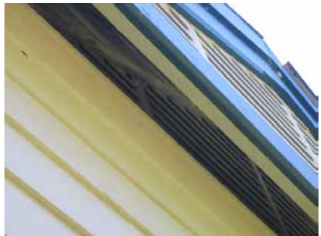
View of the double layer of louvres at the gable.
