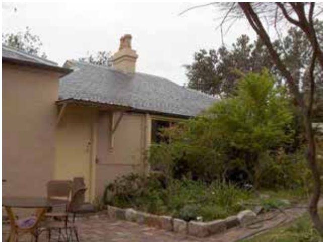
The west Assistant Light Keepers Cottage looking from the south east with the 1857 work with its filled in verandah on the right and the hipped roof 1878 extension on the left. October 2006.
