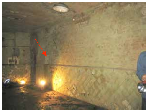
The west wall of the Engine Room. There are recesses in the brickwork for lamps (arrowed) and at the left side is the entry to the coal chute.
