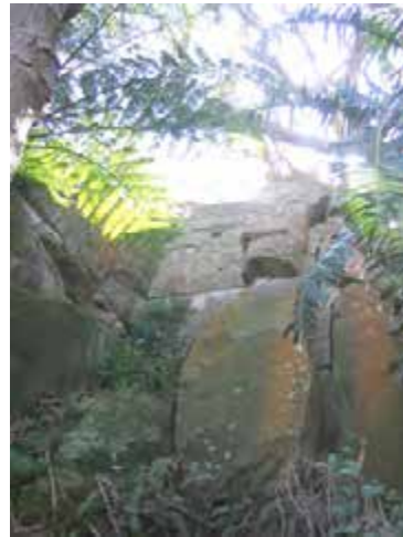
View of the rifle walls above pathway, between Constables Cottage and Cobblestone Road.
