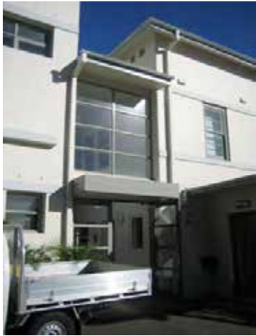
View of the front (west) entrance of building. The addition to the building is on left in the picture. Glazing of the windows above door is fixed, precluding natural ventilation.
