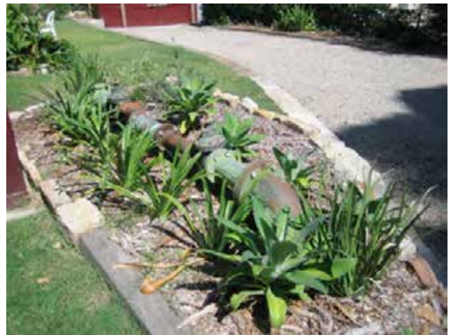
View of the front yard with major water supply installation. It is not known what this service is and where the pipes go.
