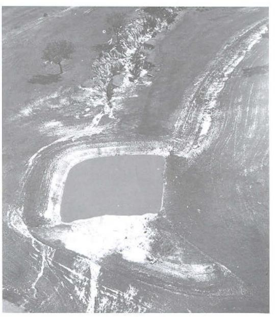
A control dam has been installed near the headwall of this gully. Any overflow from the dam is diverted from the gully, thus preventing further erosion.
