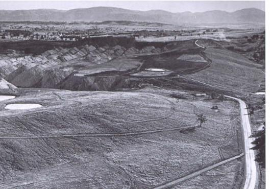
More than 100 years of mining operations left a 15 hectare waste dump at Captains Flat, near Canberra. The eroding dump sent toxic matter into the Molonglo River and threatened the viability of Lake Burley Griffin. Following a Federal/State agreement the ravaged area was re-shaped and covered with rock and clay. The Soil Conservation Service then moved in to revegetate the entire area with grass and clover. The resulting 'new' landscape is shown in this photograph.
