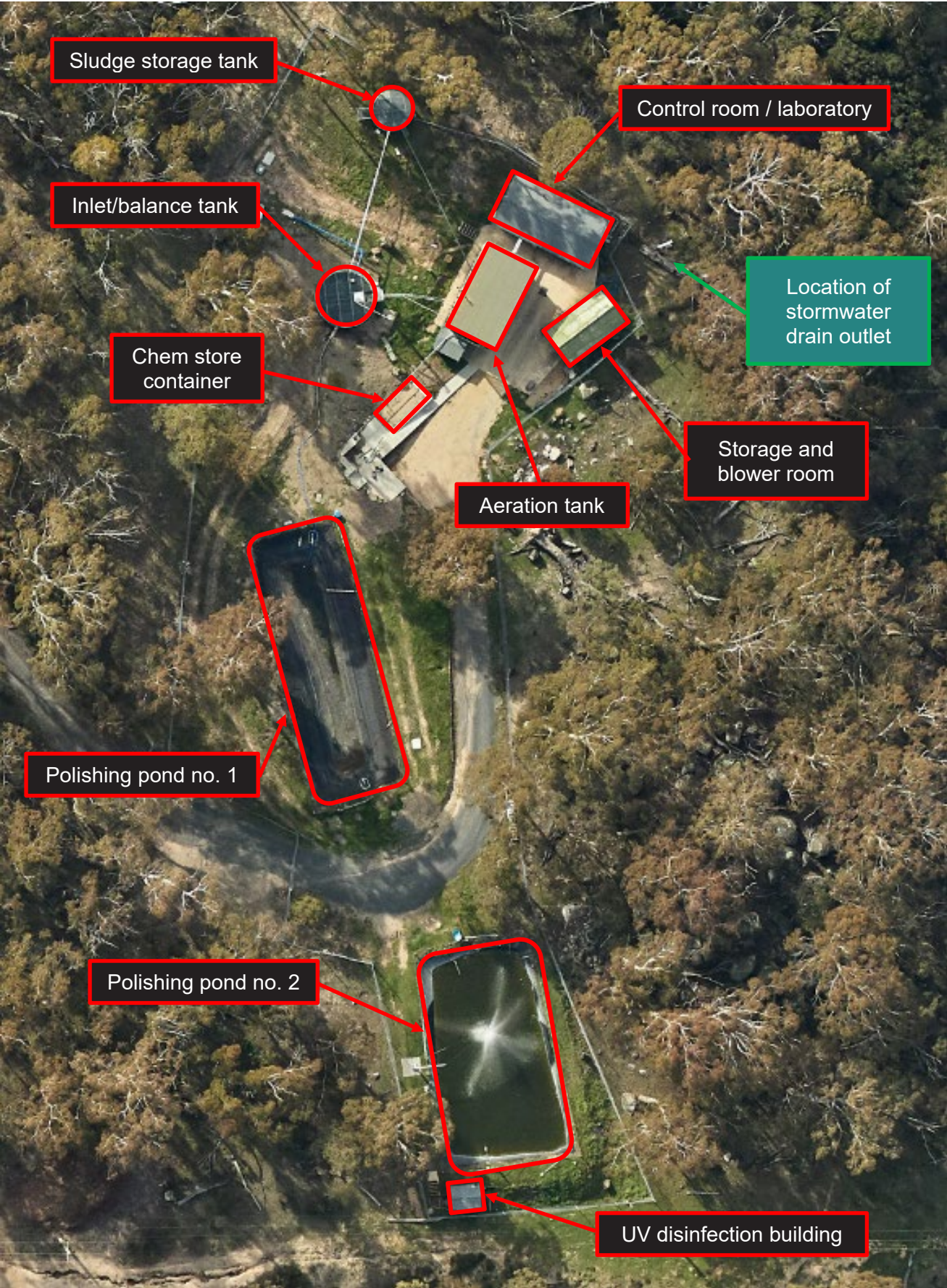
Figure 3 Aerial photo of Sawpit Creek Sewage Treatment Plant.
