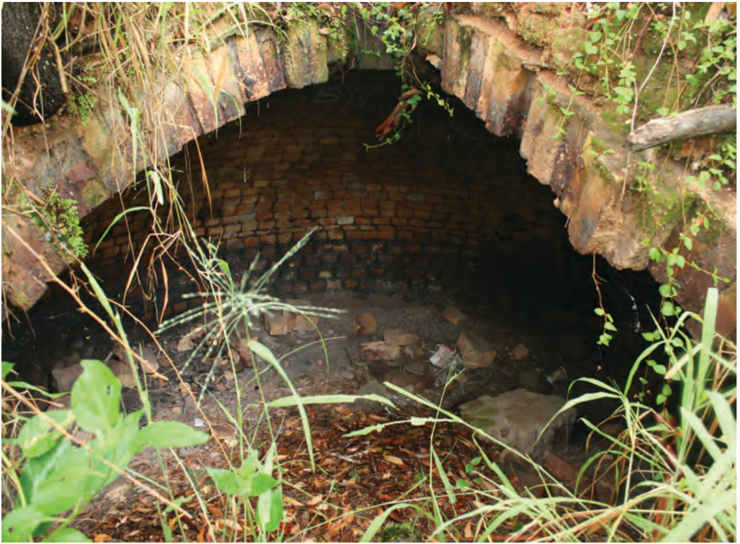
Photo: Klondyke Coke Ovens (Department of Natural Resources and Mines (Qld)).
