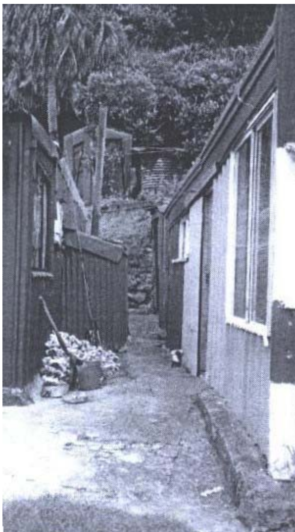
Figure 29 Concrete slab floor edges and walkways
