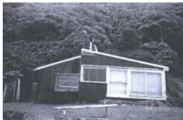
Figure 27 Cabin showing heating flue.
