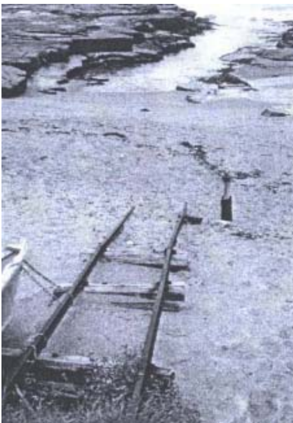
Figure 26 Boat slipway to channel.
