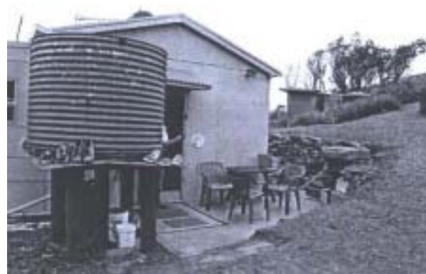
Figure 61 Cabin showing outdoor area, water tank and barbecue.
