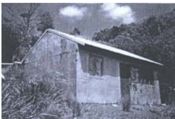
Figure 54 Iron-clad cabin, South Era valley.
