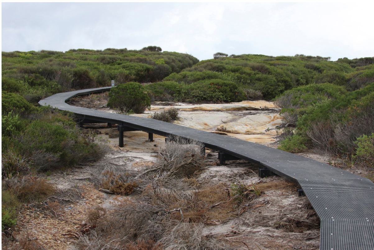
Photo 10 Boardwalk installed on the Coast Track, Royal National Park. David Croft/DPE
