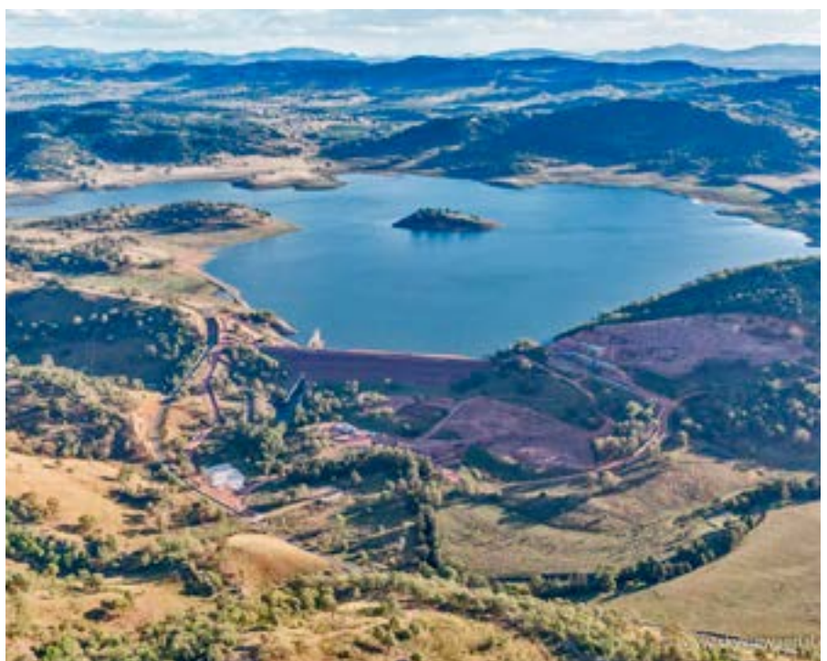
Chaffey Dam, Tamworth. WaterNSW.
