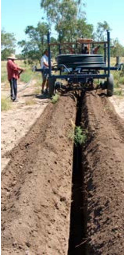
Installing underground waterpipes to save water. DPIE.
