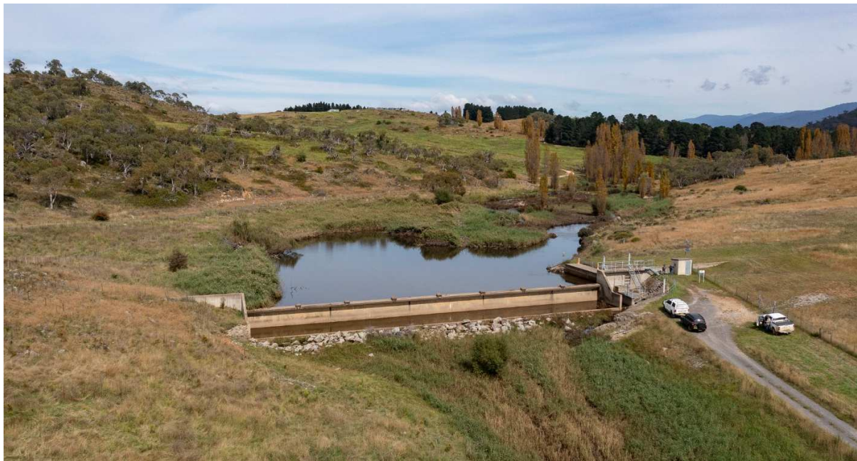
Figure 15: Mowamba Weir with no overtopping flow
