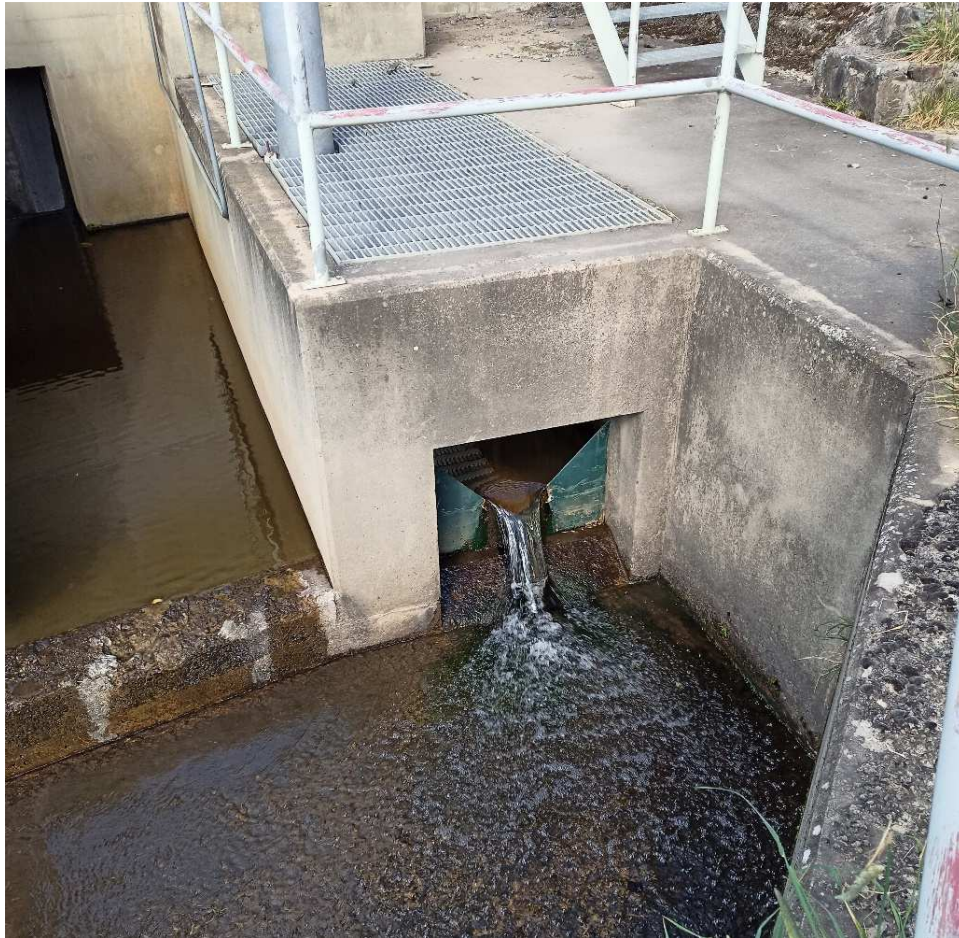
Figure 16: Mowamba Weir BPF outlet, 20 February 2022
