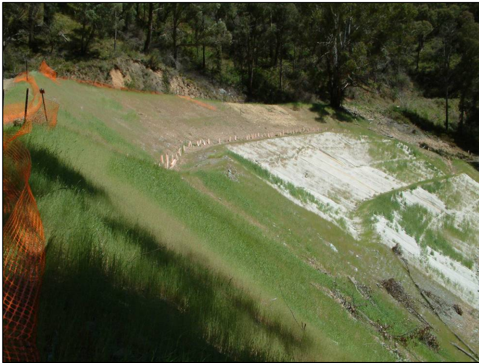
Figure A5.2.1 Sterile Rye Corn on the T2 Dogleg former Snowy site – Early February 2006. Foreground areas were located on thin soil, rear areas on rock spoil.
