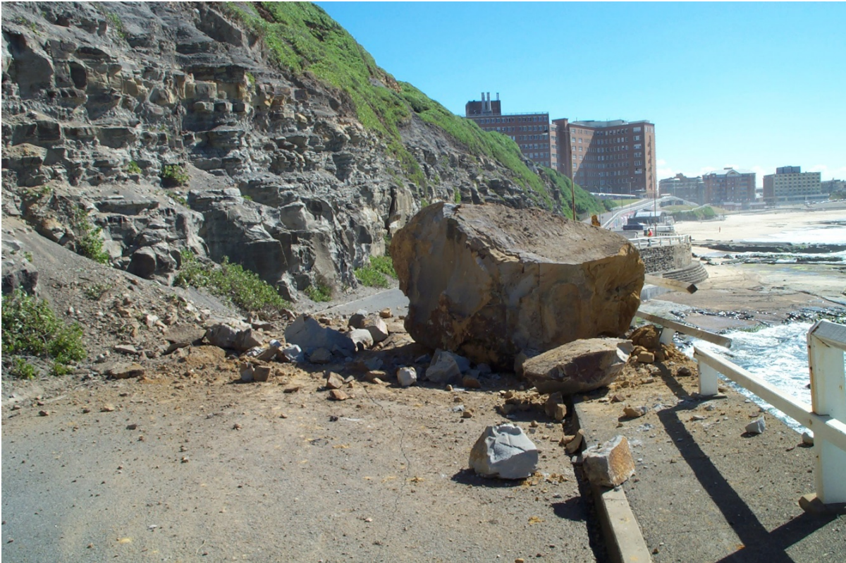
Figure 6 Rock fall from coastal cliff, Newcastle October 2002 (Photo: DPIE)
