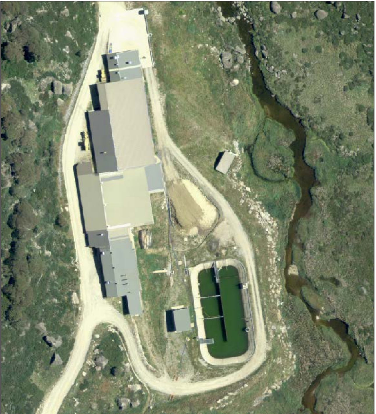
Figure 4 Aerial photo of Perisher Valley Sewage Treatment Plant
