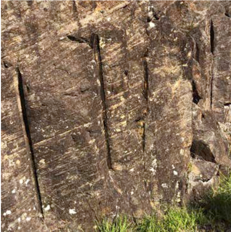
Figure 3.9: Jumper bar scars on a sandstone rock face on Devines Hill. (Photo: Richard Mackay, Mackay Strategic Pty Ltd, 2018)
