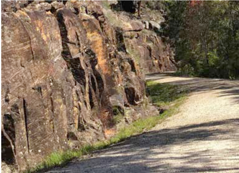
Figure 3.11: Constructed drain along inboard side of road, Devines Hill.
