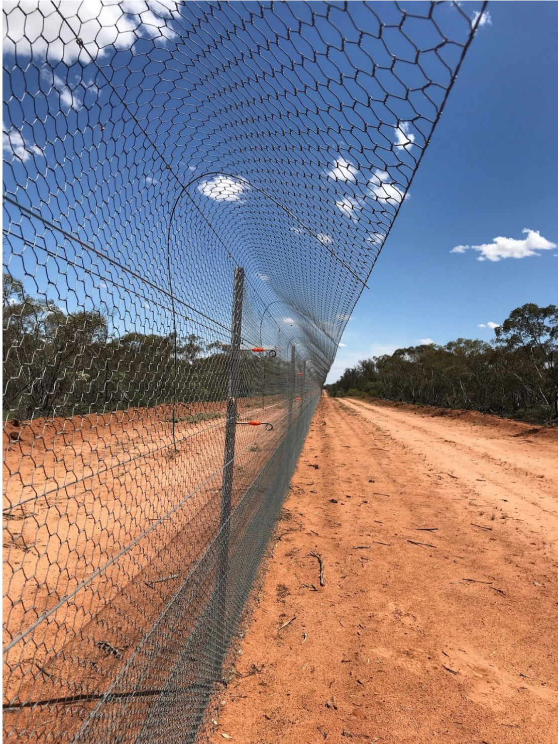
Figure 4.3 Predator proof fence at Mallee Cliffs National Park, NSW. (Source: NPWS)
