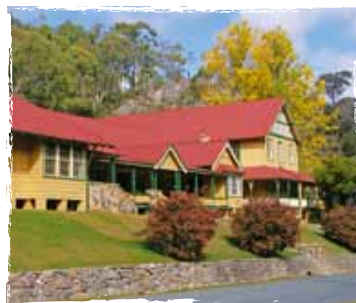
Caves House. Photo: A.Baker/OEH
