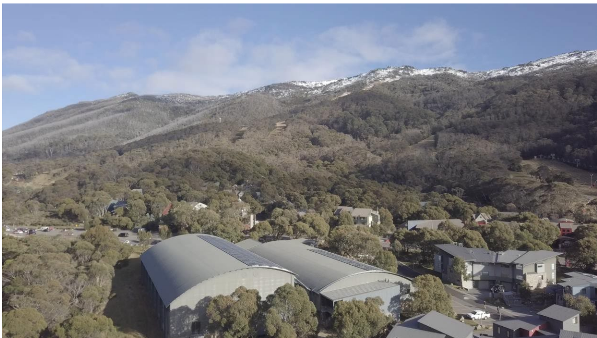
Figure 21 Solar panels on the Thredbo Leisure Centre
