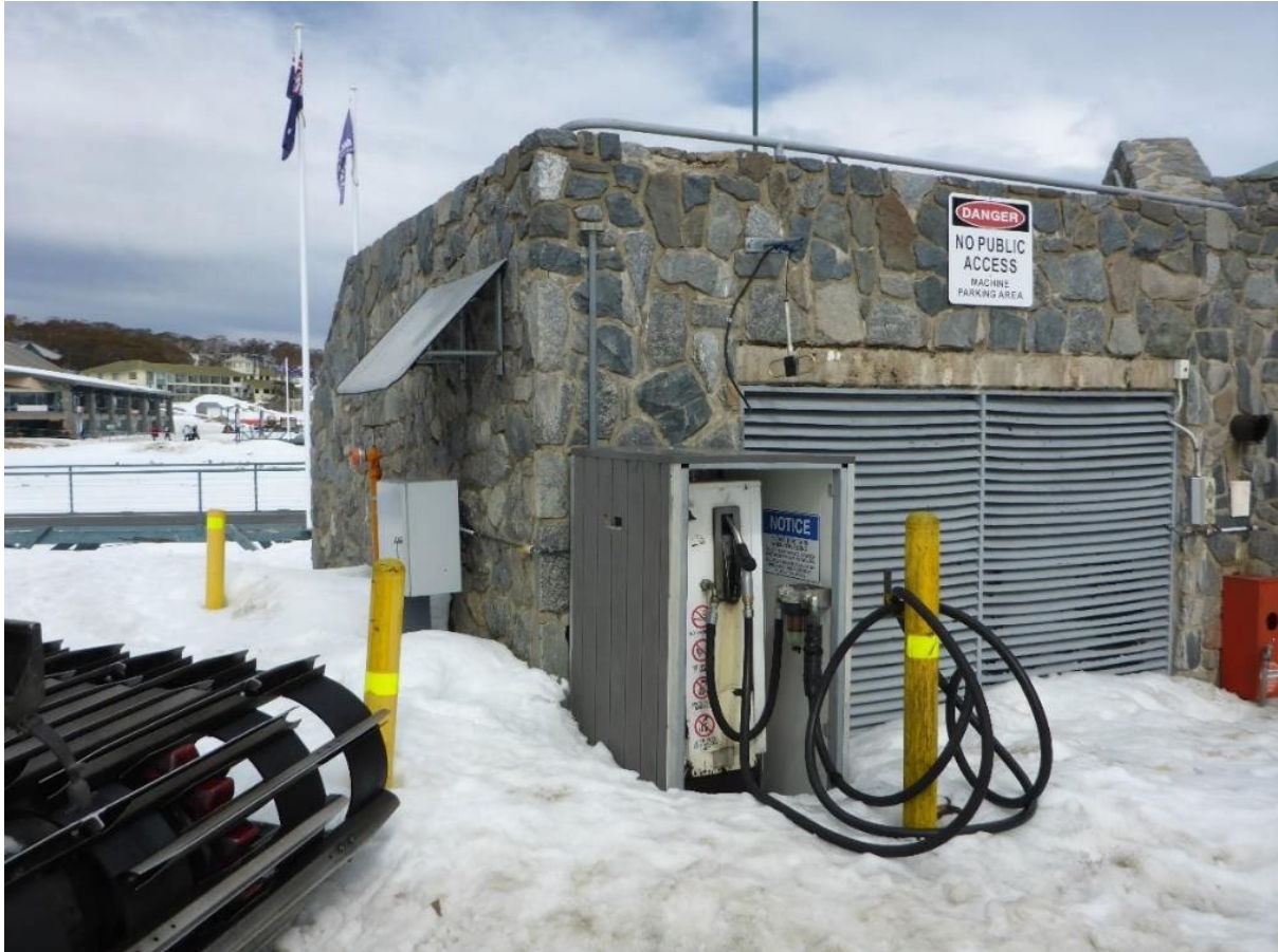
Figure 20 Snow mobile refuelling station, Perisher loading dock
