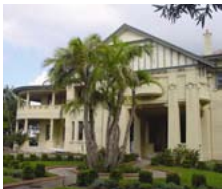
59 : Babworth House after its adaptation for apartments.
