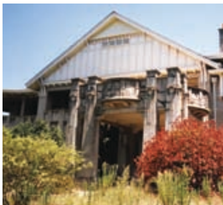
60 : Babworth House prior to adaptation.
