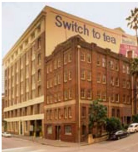
71 : The Bushells Building with its repainted façade and reinstated signage.
