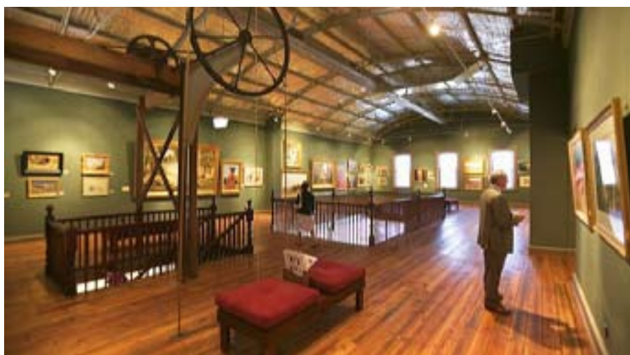
82 : The original curved roof has been lined, while still exposing the significant 1889 light metal truss.
