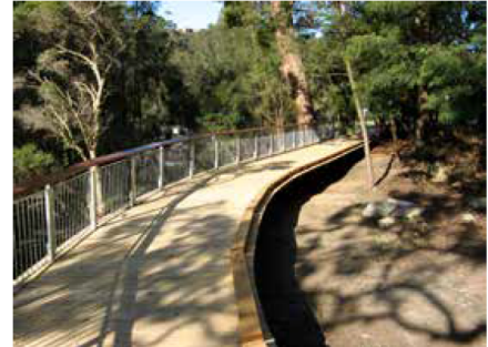
Steel frame and timber deck boardwalk at the Weir Precinct, Lane Cove NP
