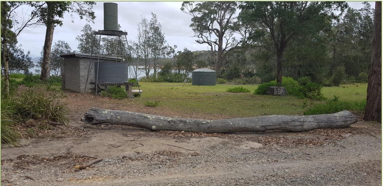
Figure 27: Yellow Rock precinct amenity building - proposed site for new wastewater treatment unit and solar system
