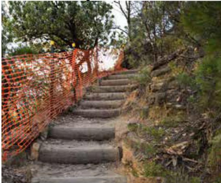
1200 long half rounds are typically used in the Blue Mountains
