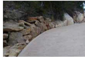
Breadcrumb oxide colour used at Three Sisters Walking Track, Blue Mountains NP
