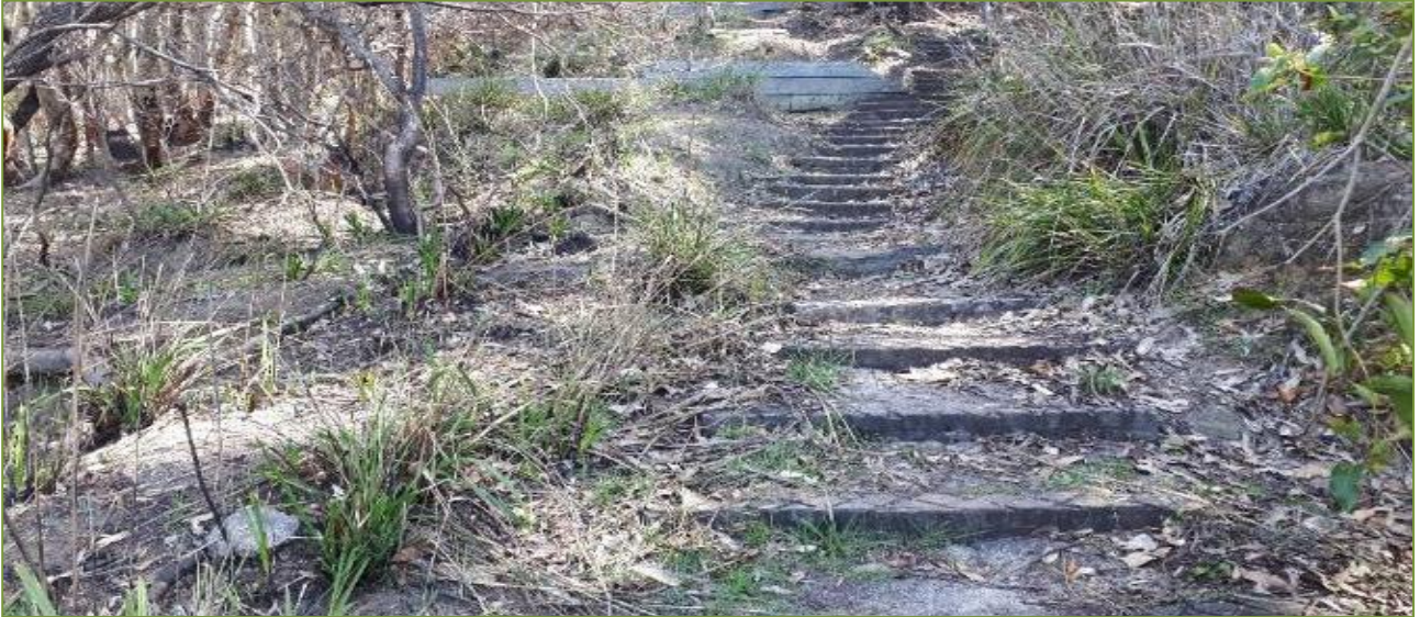
Figure 7: Example of timber stairs
