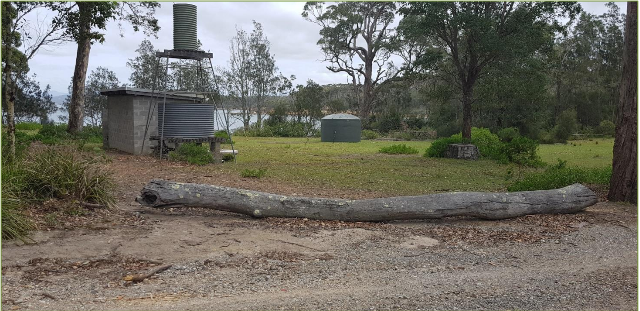
Figure 27: Yellow Rock precinct amenity building - proposed site for new wastewater treatment unit and solar system
