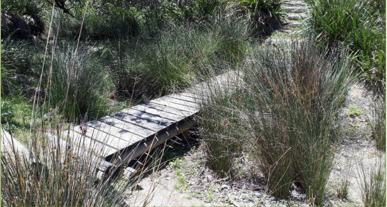
Figure 12: Example of footbridge at Richmond Beach
