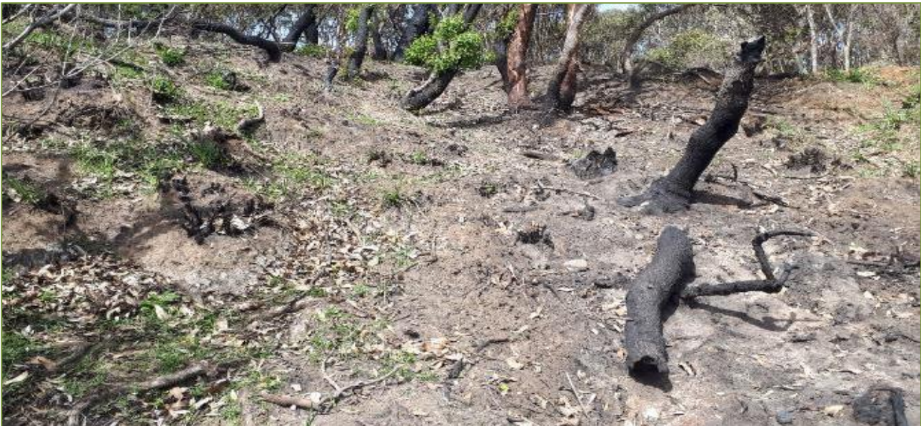
Figure 15: Eroding slope near Depot Beach
