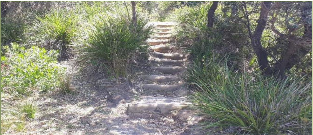
Figure 9: Timber stairs at Honeysuckle Bay requiring maintenance
