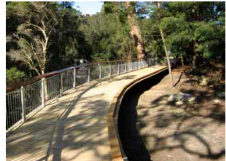
Steel frame and timber deck boardwalk at the Weir Precinct, Lane Cove NP
