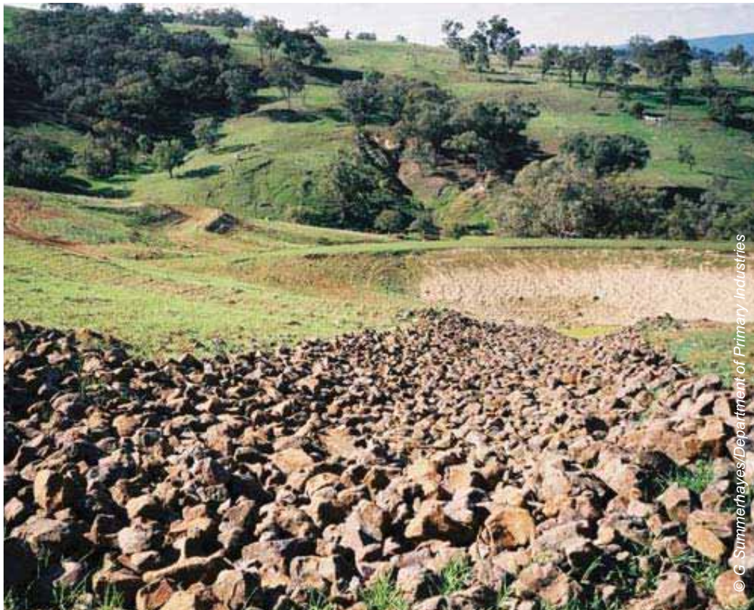
Figure 6.2 Rip-rap rock waterways conveying runoff to a sediment basin
