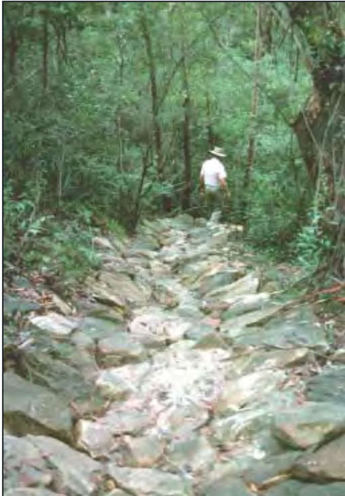
Figure 5.4 A rock-lined waterway
