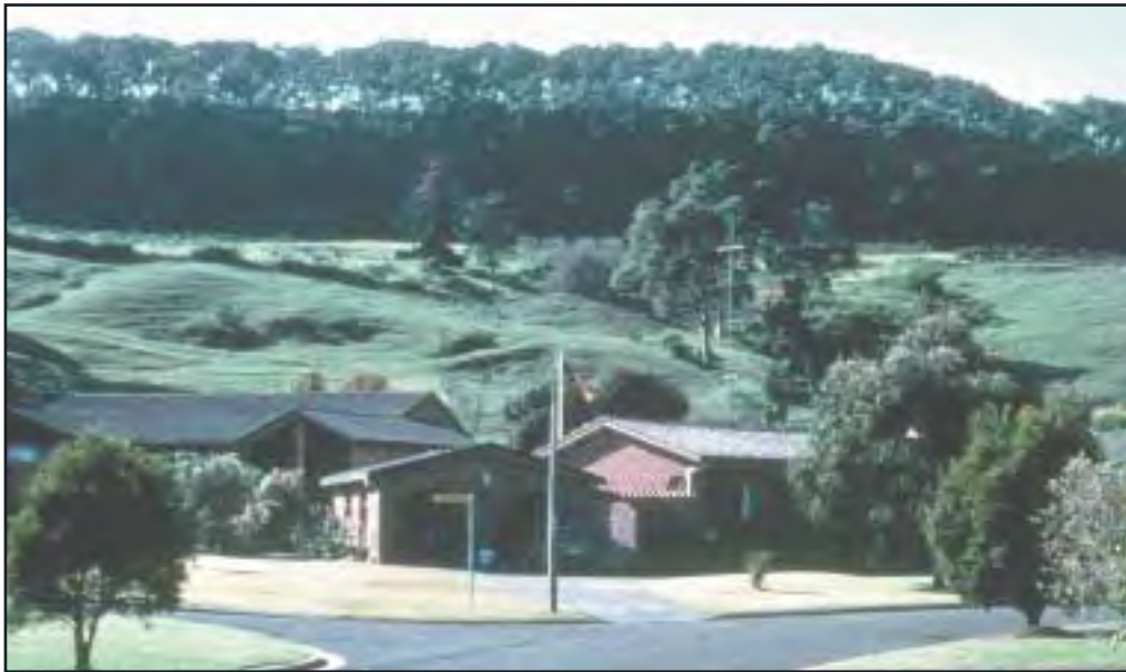
Figure 3.1 Landslip in the Picton area of New South Wales.
