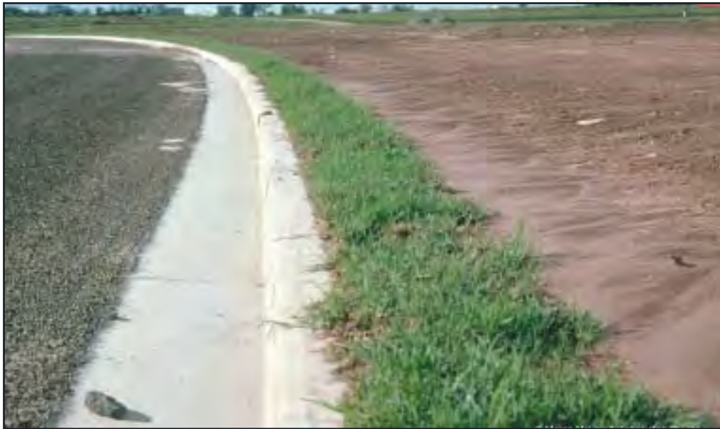
Figure 6.12 A kerbside turf strip showing sediment stored in the area above the filter.
