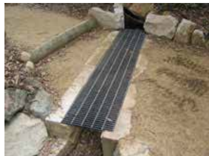
Cross drain with fiberglass mesh grate (Wentworth Falls, Blue Mountains National Park)
