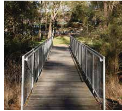
Steel frame and timber deck bridge at Lane Cove NP
