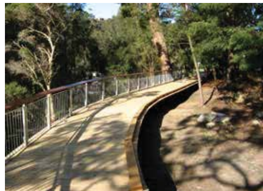
Steel frame and timber deck boardwalk at the Weir Precinct, Lane Cove NP
