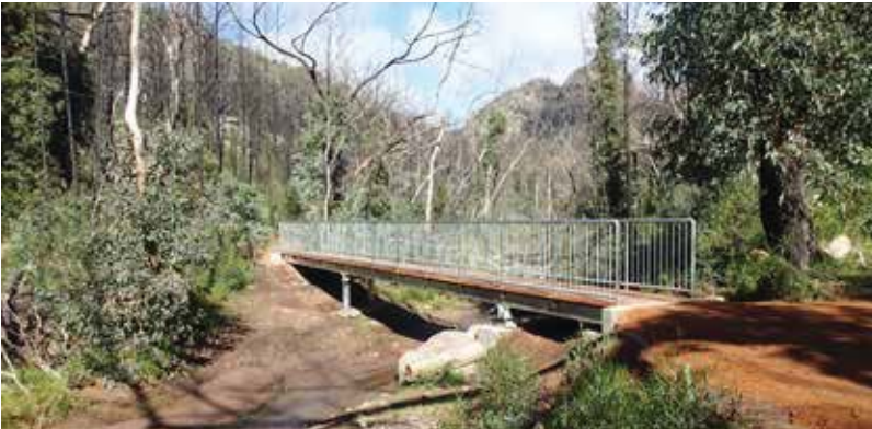
Steel frame and timber deck bridge at Warrumbungle NP
