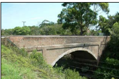
Local heritage A good example of a brick arch bridge associated with the early 20 th century electrification of the Illawarra rail line – Rail bridge, Thirroul , circa 1920s
