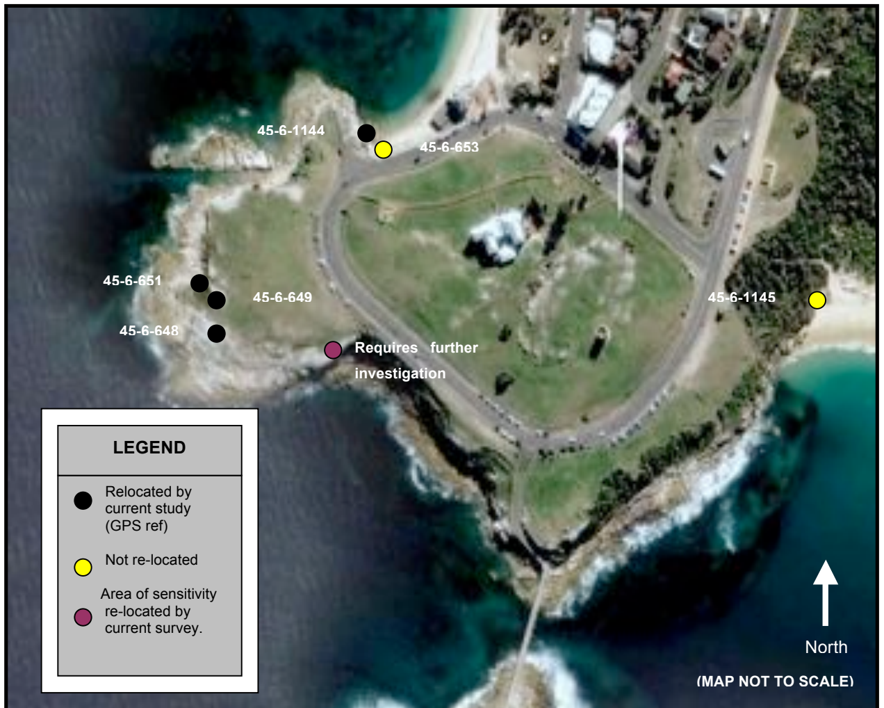
Figure 4.5: Aboriginal site locations La Perouse Headland. (Note: Campbell's grid reference is the same for -649 and -650 and 45-6-650 was not relocated. Refer to Table 4.3)
