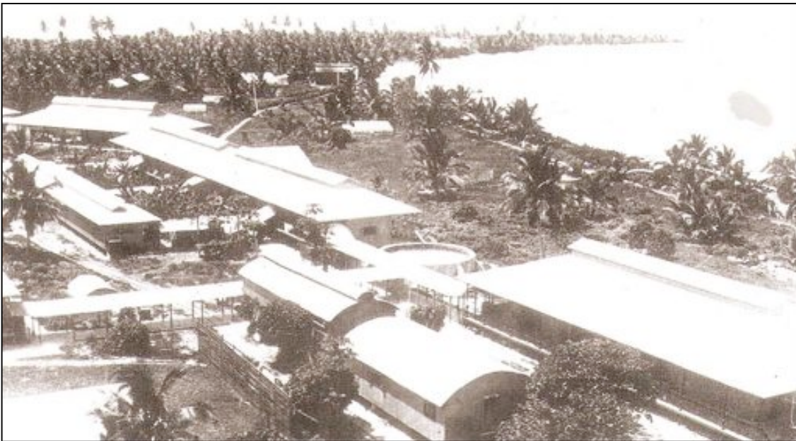
Figure 6.19: Cable Station Cocos Island .nd. Photograph reproduced from Airey E 2005.
