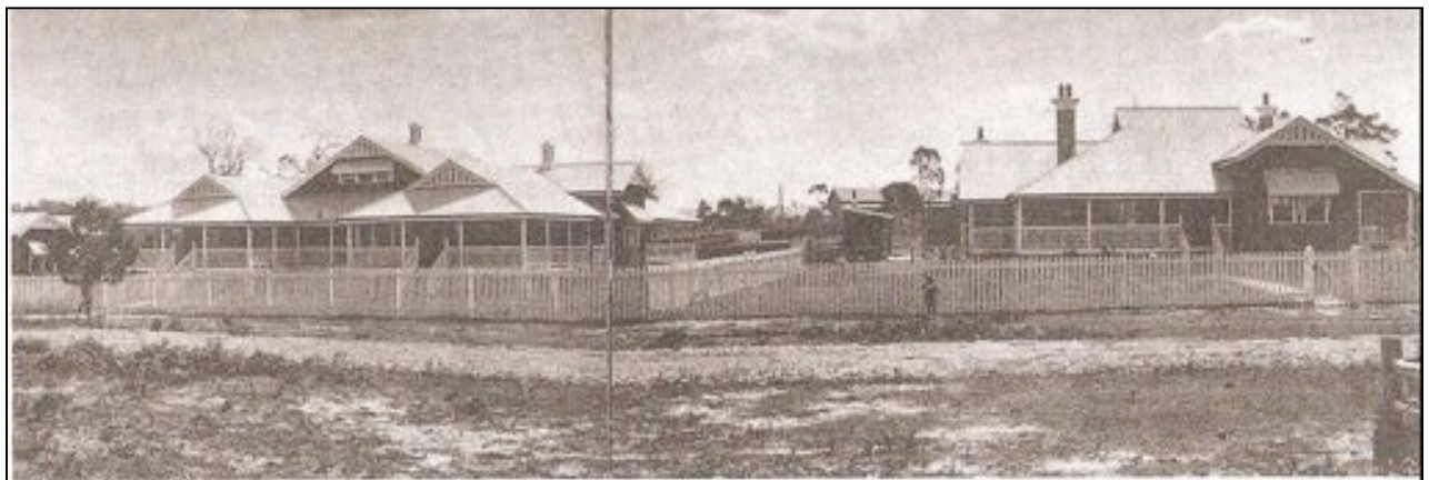
Figure 6.14: Cable Station at South Port, Adelaide. The building on the left contained living quarters for several operators and the matron of the training school which was based at the station. The second building housed the manager's office, operations room and probationers quarters. (Reproduced from Miller M c1992: 19 [MLF384.10994])
