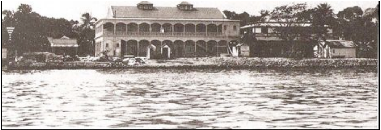
Figure 6.13: Cable Station at Suva, Fiji c1924. Photograph reproduced from Scott B R 1994.
