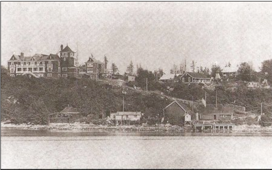
Figure 6.15: Bamfield Cable Station and wharf at Bamfield Creek, British Columbia, c1918. On the hill to the left is the main building which housed the manager's office, operating room, bachelors' quarters, mess hall and telegraph room. Married staff cottages are on the right and in the centre front is the engine room. Photograph reproduced from Miller M c1992.
