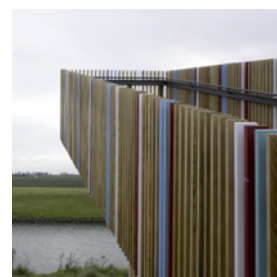
T-1 Timber Batten Screen painted + left to weather grey (alternating) steel frame behind
