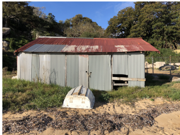
B Station Beach Shed
