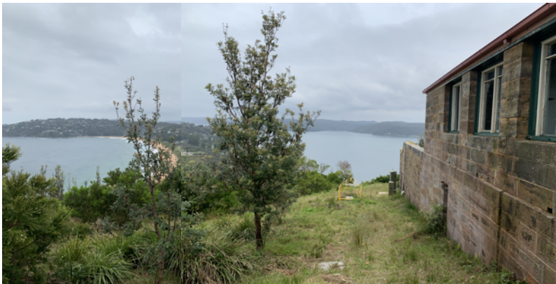
E View Looking Down Hill Towards Site
