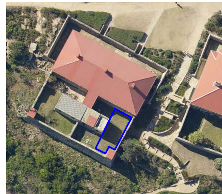
04 Aerial View of Site Storage Area in Assistant Lightkeeper's Duplex nts
