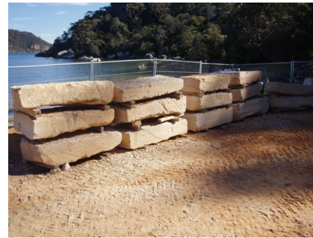
Photos of the Construction Staging Area During 2007-2015 Trail Upgrade Works
