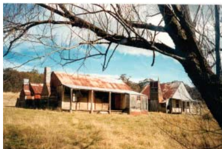
Figure 3.23 Coolamine Homestead the centre of a large pastoral holding (Southwell House, left), from the first grazing period. 37
