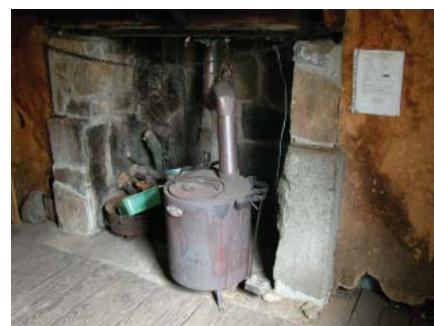
Figure 3.61 Slow combustion stove within stone lined fireplace at Mawson's Hut (caneite lining adjacent).
