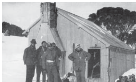
Figure 3.34 Mawson's Hut, 1963, with cross-country skiers en route between Kosciuszko and Kiandra. 47
