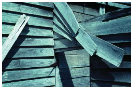
Figure 9 Detail of timber fabric of Gooandra Homestead.
