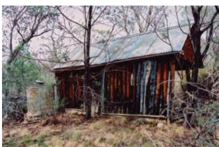
Figure 3.68 Rugman's Hut; its construction possibly associated with brumby running in KNP. 57
