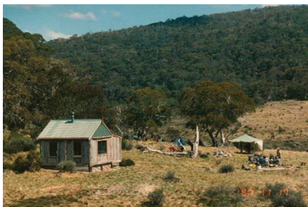
Figure 3.66 Former Burrungabuggee Hut, built as a trackhead facility, nearby to the site of Constances Hut. 62
