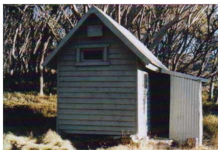
Figure 3.29 SMA Hut (Pipers Creek) built for aqueduct maintenance. 42
