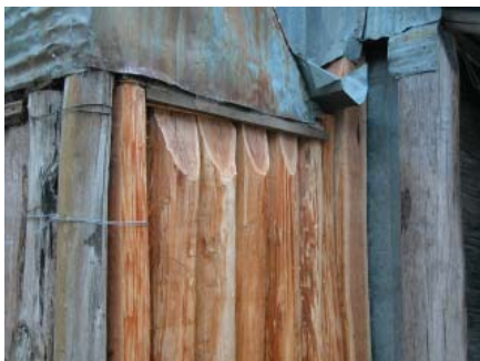
Figure 2 Chimney detail of Wheeler's Hut, after conservation works.
