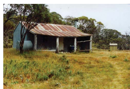
Figure 3.15 Mackey's Hut, located on the edge of a cold air drainage herbfield, Happy Jacks Plain. 33
