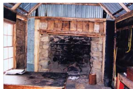
Figure 3.55 Interior of Wheeler's Hut, showing timber pole construction.
