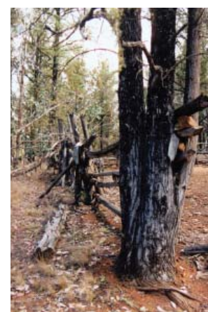
Figure 2.3 Holding pen for travelling stock, traditional vernacular construction using available materials (surrounding saplings), constructed latter part of twentieth century (c1960s).
