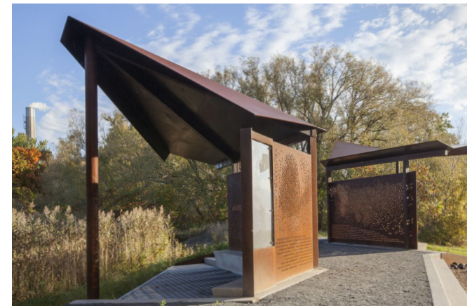
Potential for upgrading interpretation displays East Point Park Bird Sanctuary Pavilion (PLANT 1)
