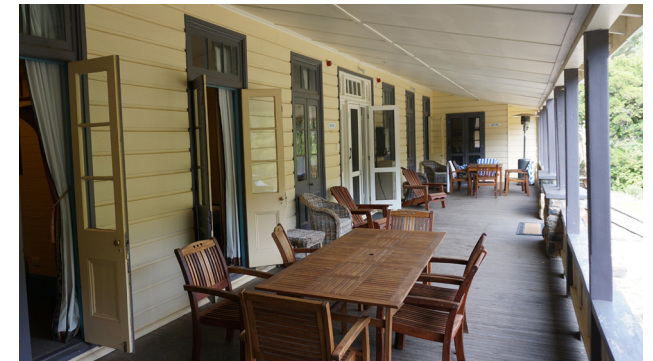
Northern Verandah and main entry Caves House 1901 wings (JPW)
