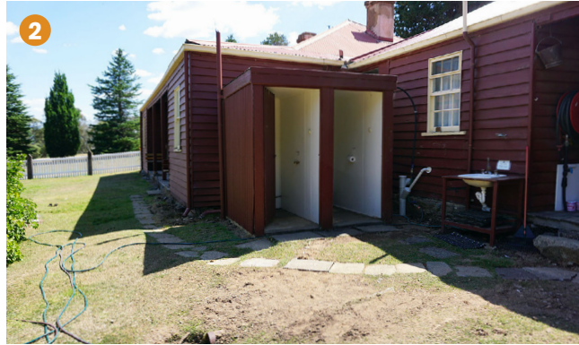
2. External toilets Currango Homestead(JPW)
