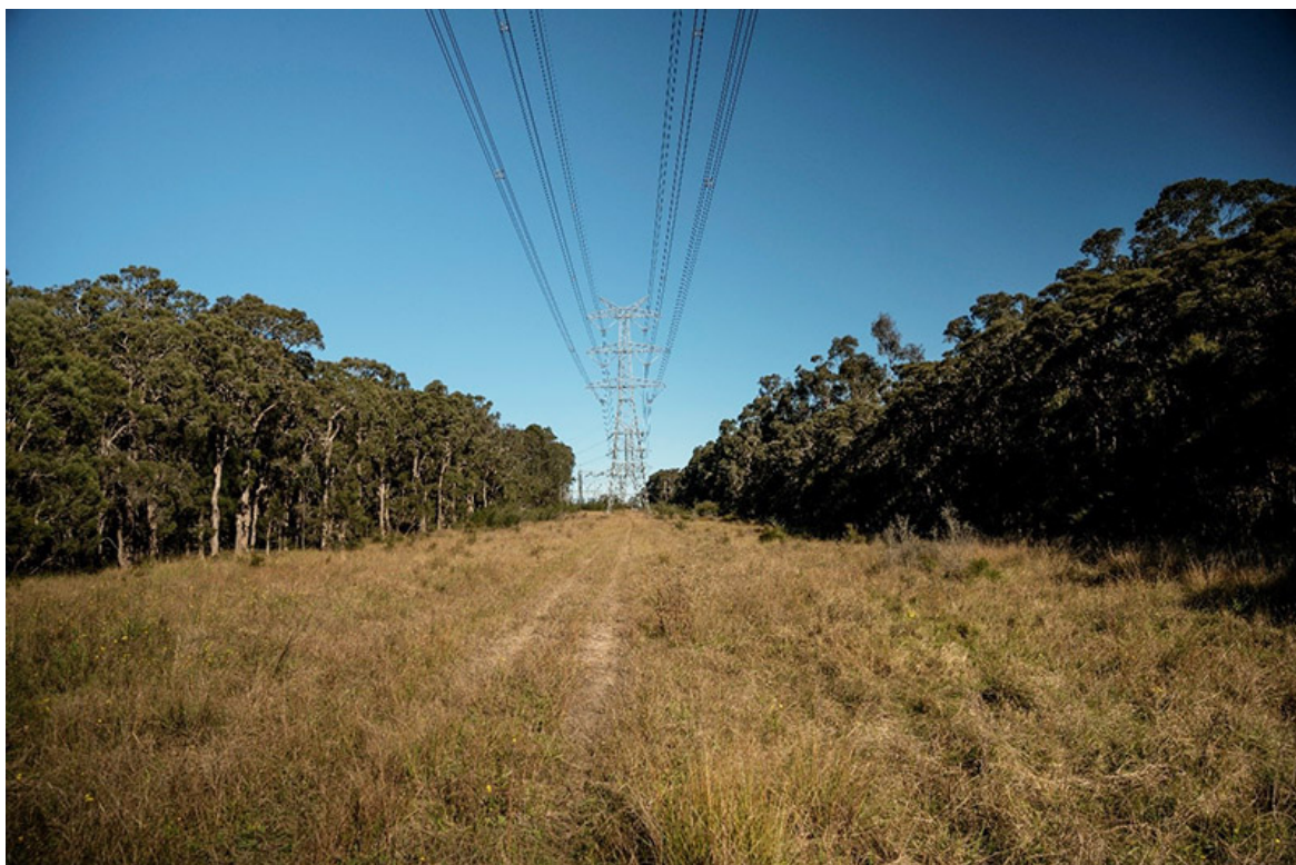
Photo 12 Cleared electricity easements, Kemps Creek Nature Reserve. Darren Roberts
