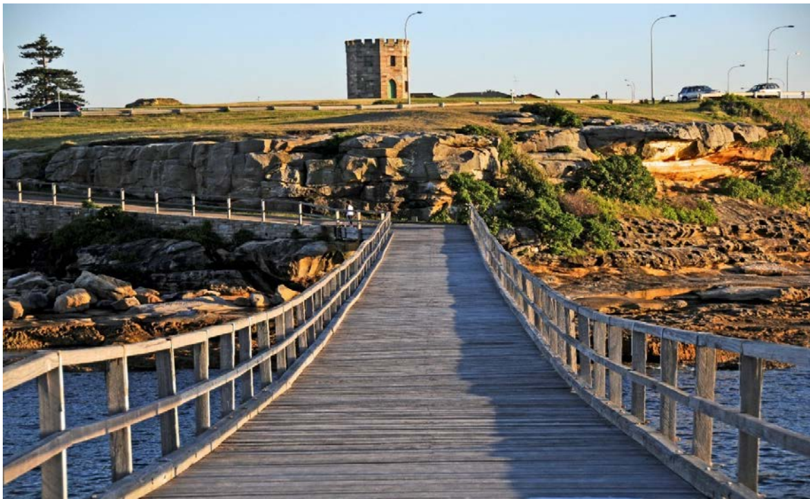
Wooden footbridge linking Bare Island to the mainland. Photo: Kevin McGrath/DPIE.
