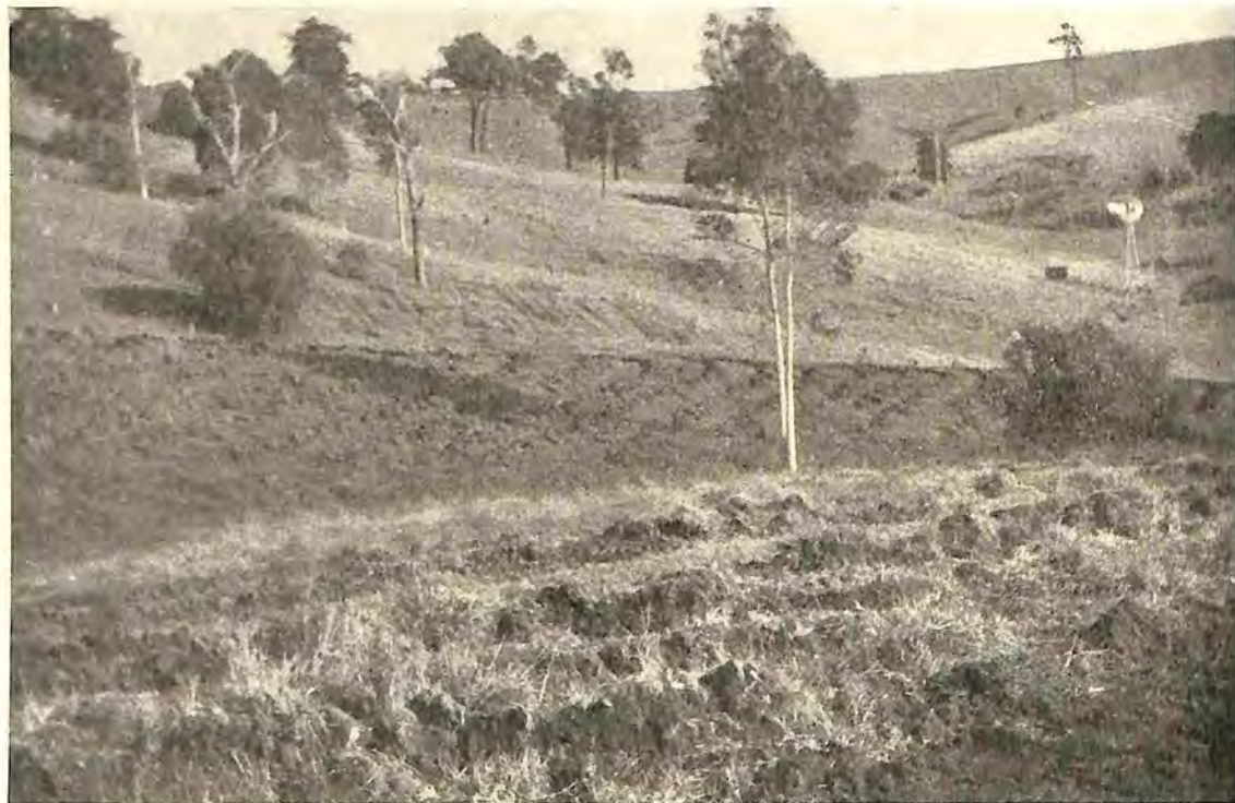
Fig. 7.—Pasture furrows used to prevent the onset of erosion and increase cover.
