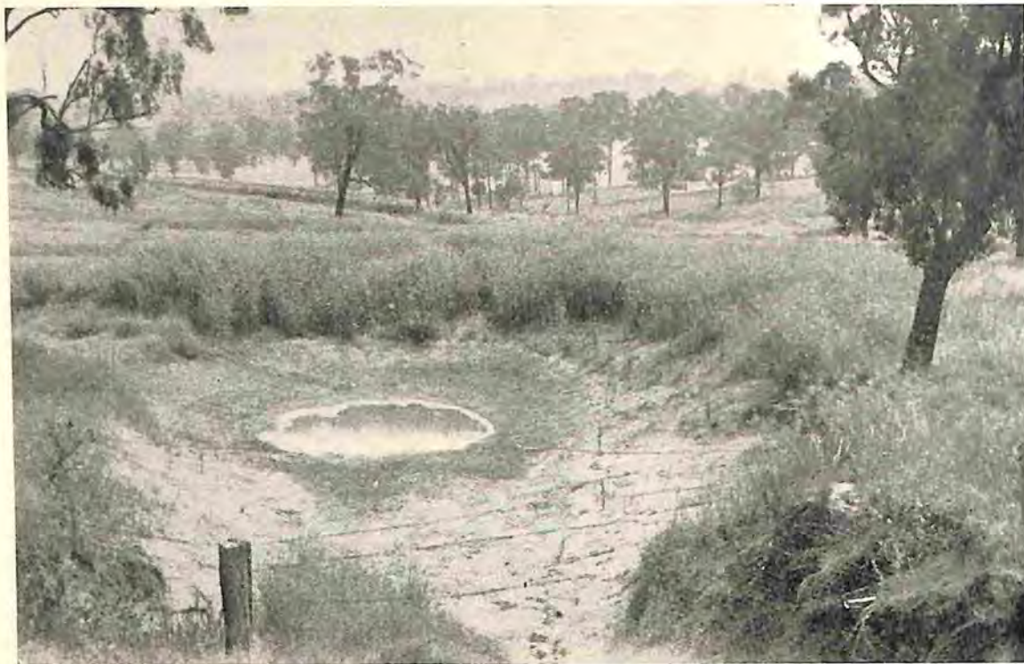
Fig. 4.—The gullied area shown in Fig. 3 after stabilisation by silt dam construction and outlet via a vegetated waterway.
