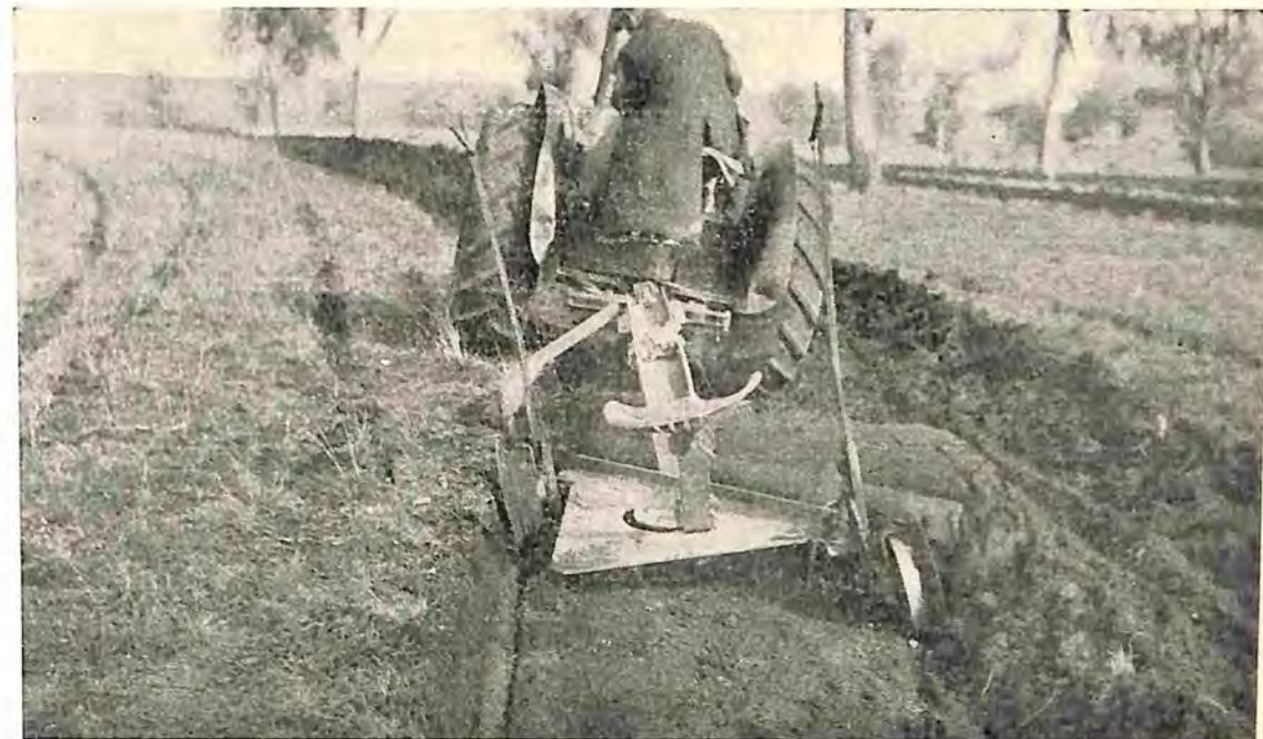
Fig. 5.—Constructing a graded bank with small plant. Cowra district.
