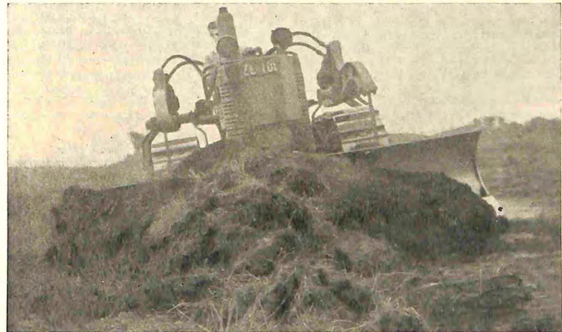
Fig. 4.—Heavy equipment preparing land for soil conservation work.
