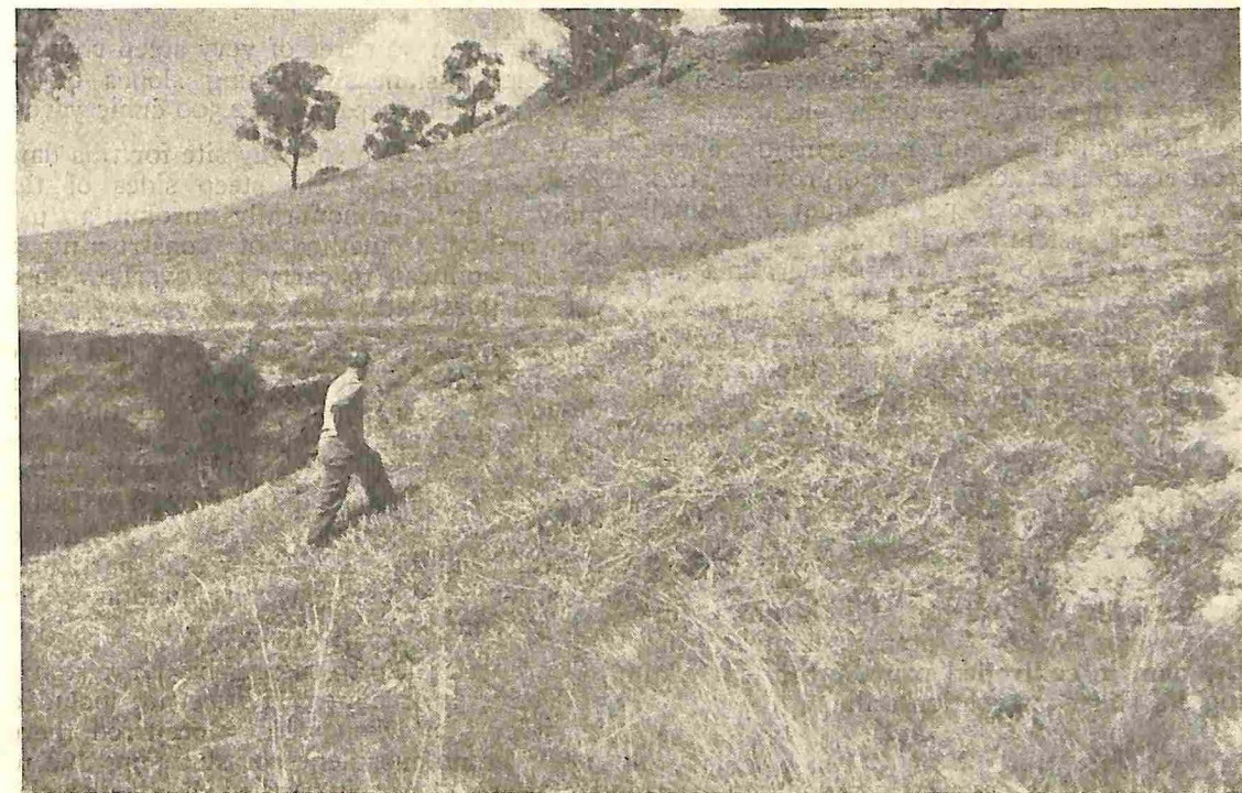
Fig. 2.—No. 1 dam spillway showing notch outlet and heavy growth of kikuyu on race.
