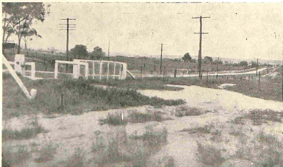
Fig. 3.—The main waterway, well established in 1950, carries a flow 9 inches deep in safety after heavy rains.
