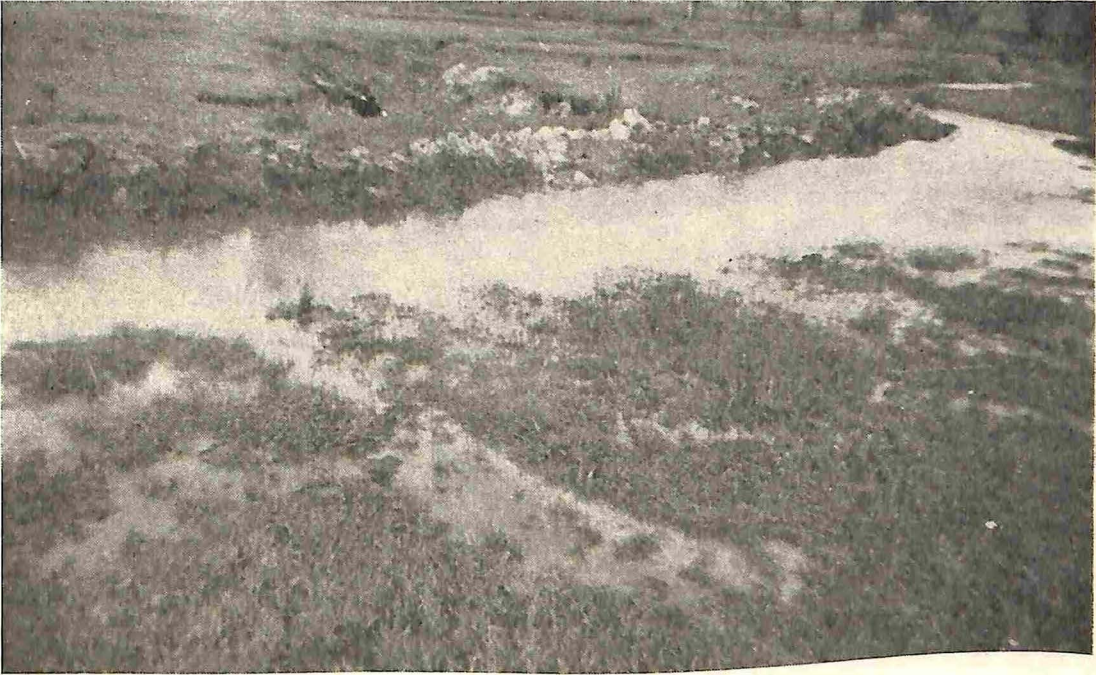
Fig. 5.—Diversion bank protecting gully head.
