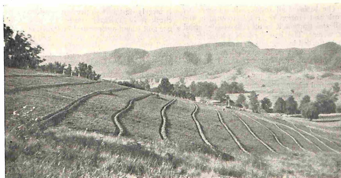
Fig. 1.—Contour furrows constructed on hilly grazing land in Kangaroo Valley. The mouldboard plough in Fig. 2 was used for construction.
