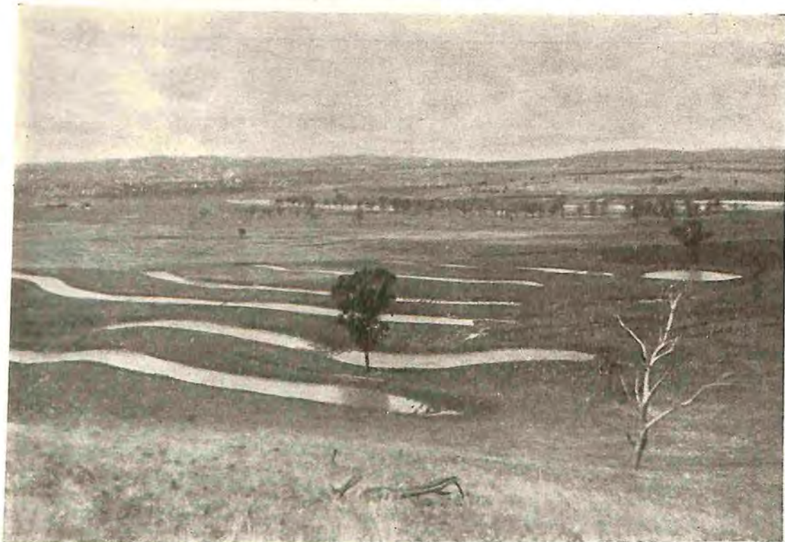
Fig. 4.—All the rainfall retained on the land after mechanical works have been undertaken.
