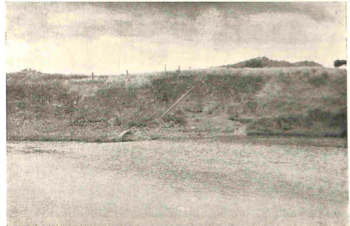
Fig. 4.—Further recent erosion 500 yards below the weir adjacent to the racecourse.
