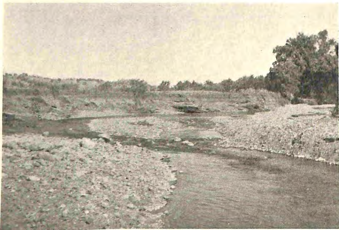
Fig. 5 —A change in the course of Hall's Creek at high flow brought about the damage to the banks shown in the background.
