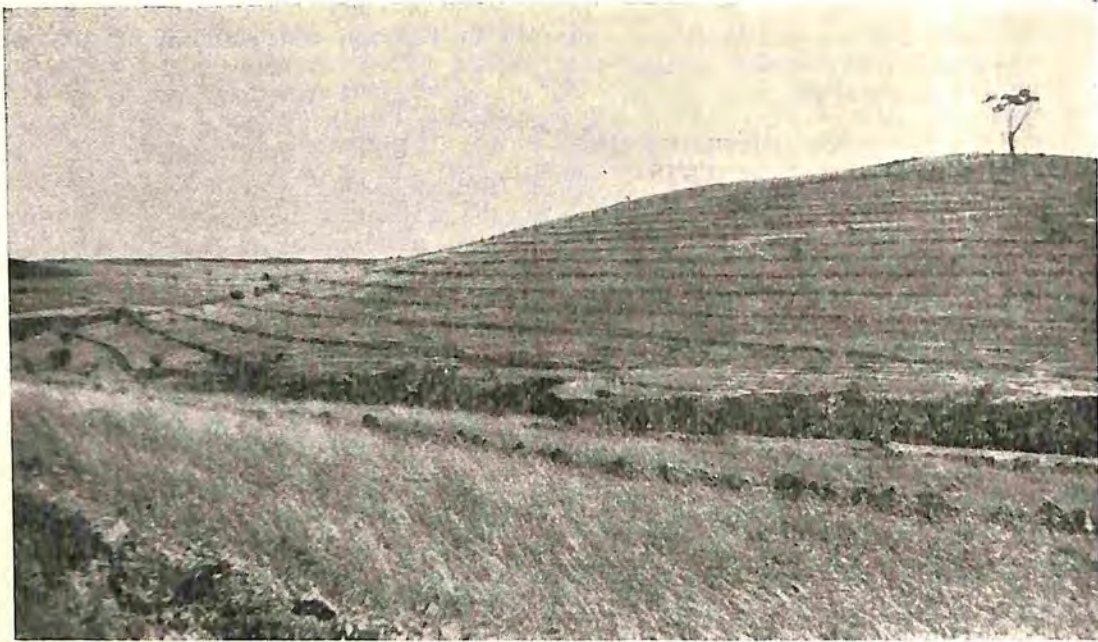
Fig. 5.—Contour furrows on eroded areas adjacent to the country killing works, Goulburn.
