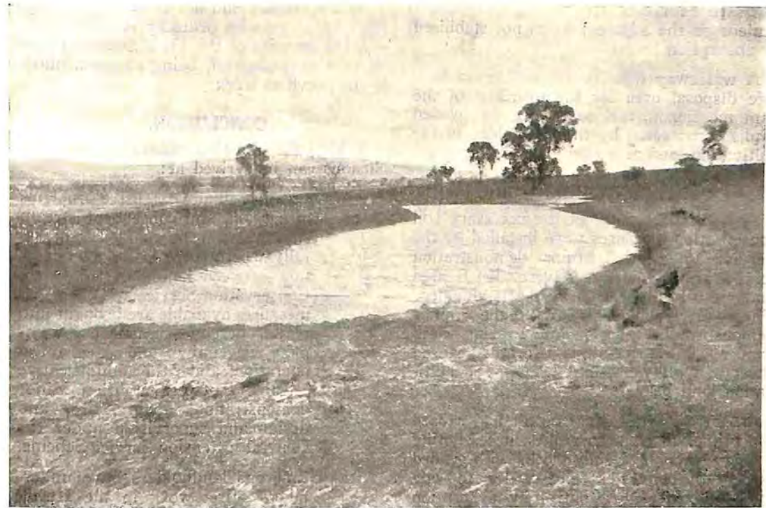
Fig. 5.—A typical absorption bank, following heavy rain. The outlet is in the foreground.
