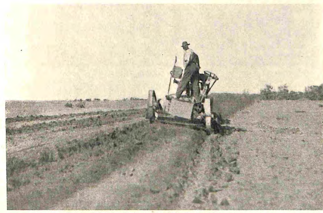
Fig. 6. —Trimming the lower side of the bank with grader-terraccer.
