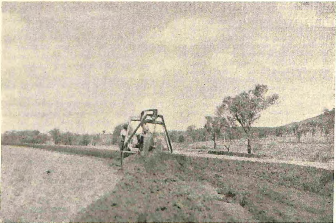
Fig. 4. —The final cut by the angledozer, forming the batter.
