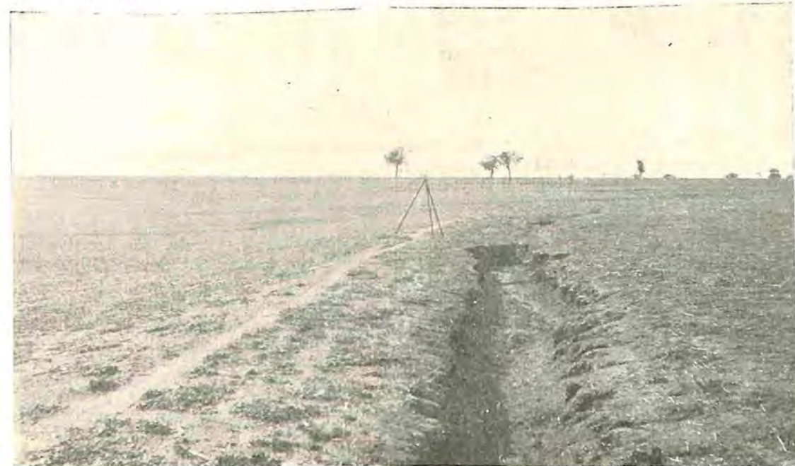
Fig. 2.—This gully formed in the bank channel because of excessive grade.
