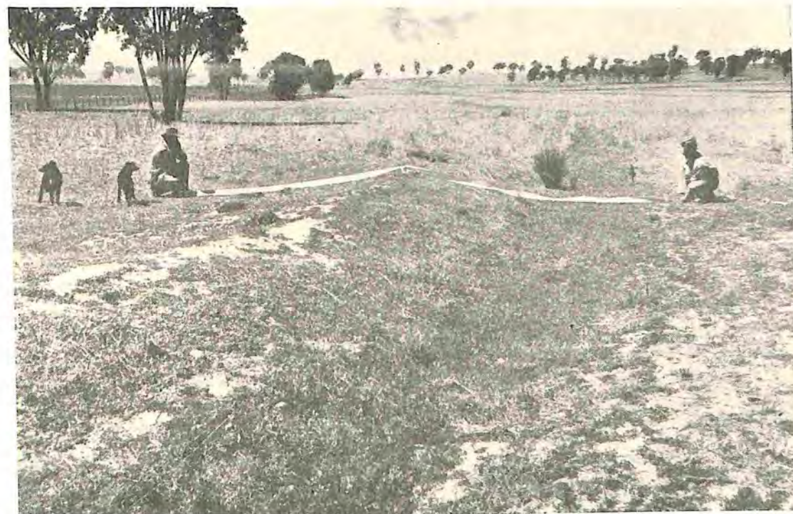
Fig. 4.—A well-vegetated diversion bank leads water to a safe outlet.
