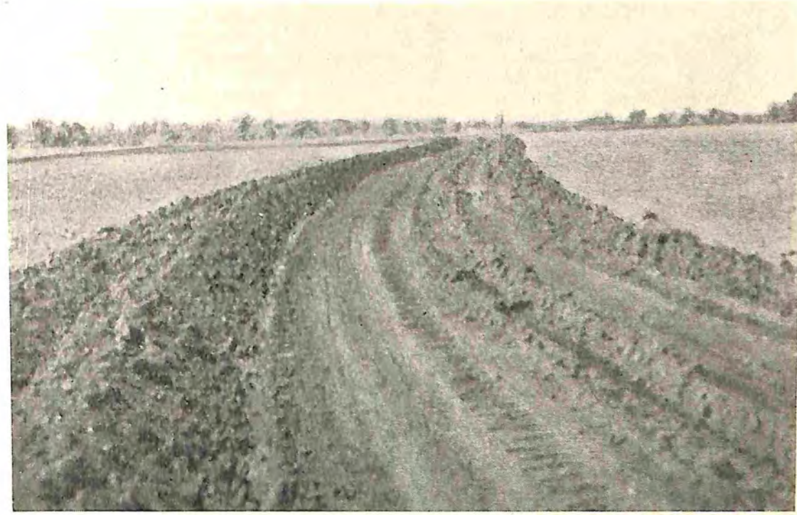
Fig. 5. —The bank and channel at completion of work by the angledozer.
