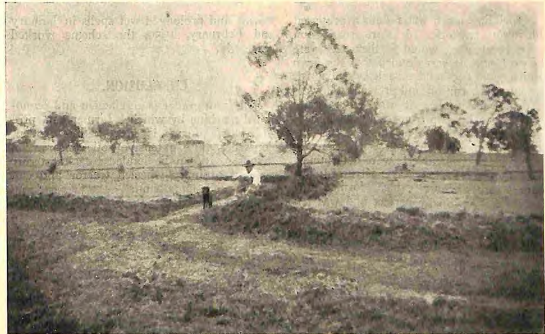
Fig. 5.—The outlet of the graded bank in Fig. 4 into a natural grassed waterway. The bank in both left and right foreground is the trainer bank of the waterway.
