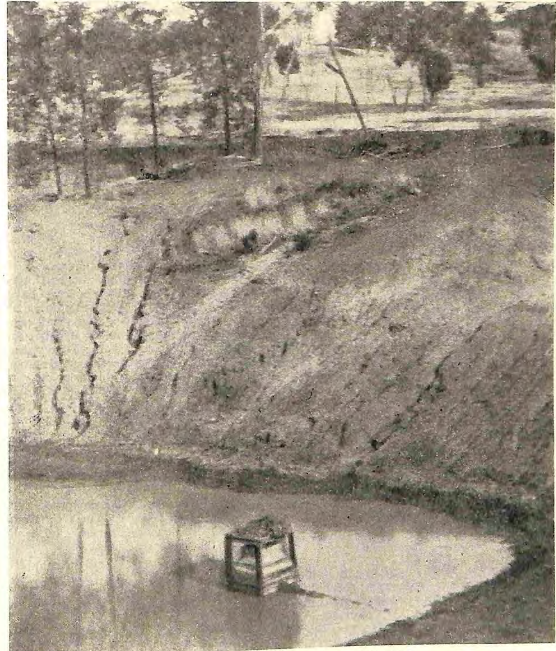
Fig. 2.—Showing inlet structure for emptying dam.
