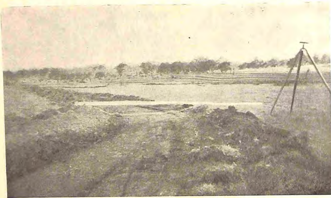
Fig. 2.—Construction of a graded bank at King's Plains.
