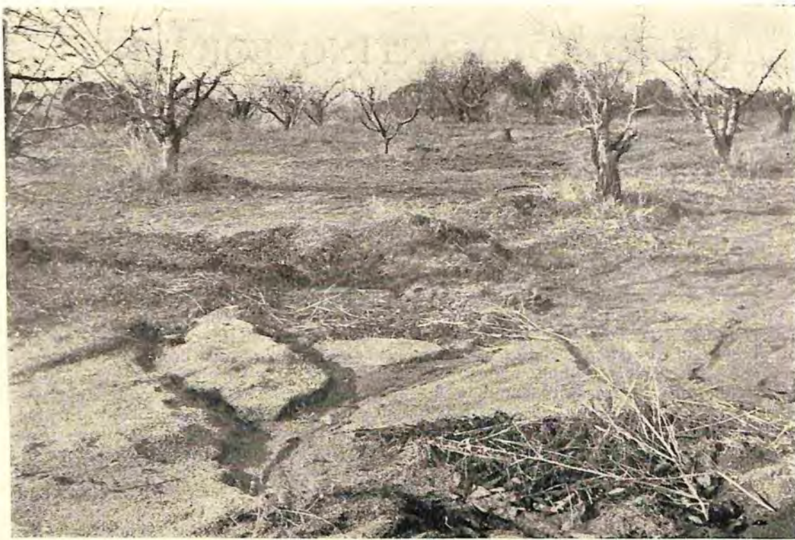
Fig. 1.—Orchard erosion. Contour planting and cultivation will prevent this occurring.
