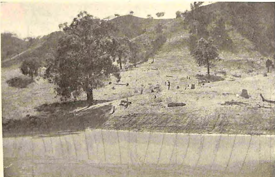
Fig. 3. —A newly constructed dam designed for the soil conservation programme. Note the steep nature of the catchment.
