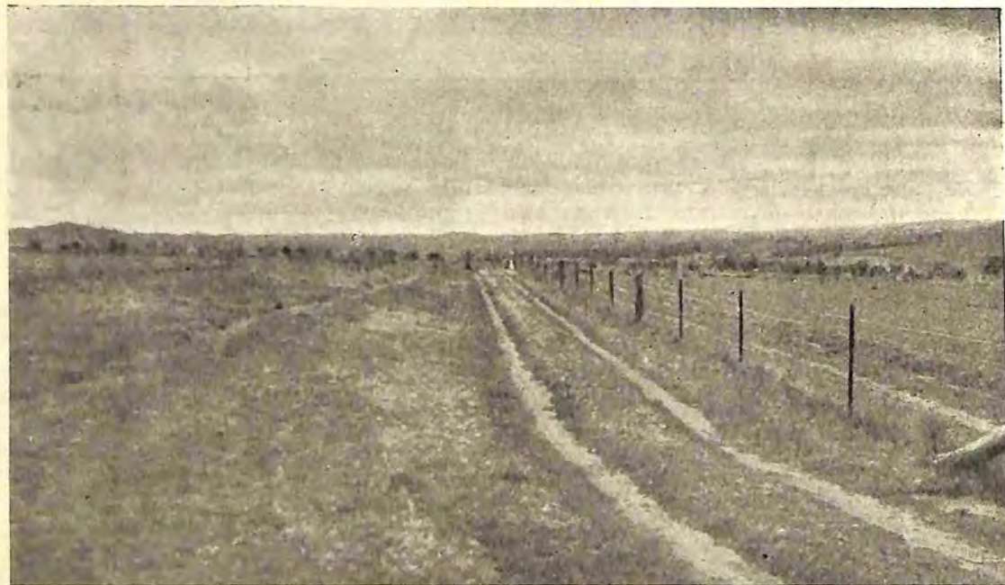
Fig. 4. —This farm road is running on the contour and the run-off water is prevented from reaching it by pasture furrows.
