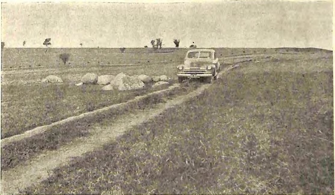
Fig. 6. —Road running along the top of a graded bank, almost a contour.
