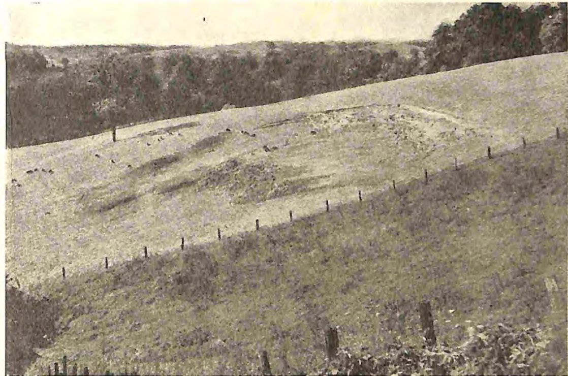
Fig. 11.—A typical earth flow showing slumping at head and bulging at base of flow. (Photo by U.S.D.A.)
