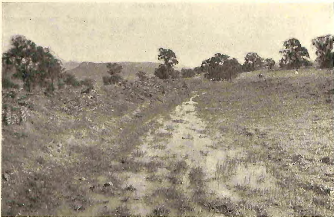
Fig. 4. —The overflow from the dam shown in Fig. 3 safely conducted along a grassed diversion bank.
